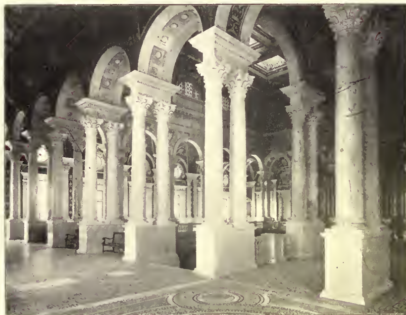
Central Corridor and Light Well
