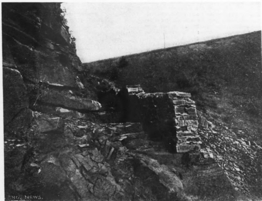
FIG. 2.—VIEW OF DOWNSTREAM FACE OF CASCADE ROCK FILL AND OUTLET OF SPILLWAY TUNNEL.
