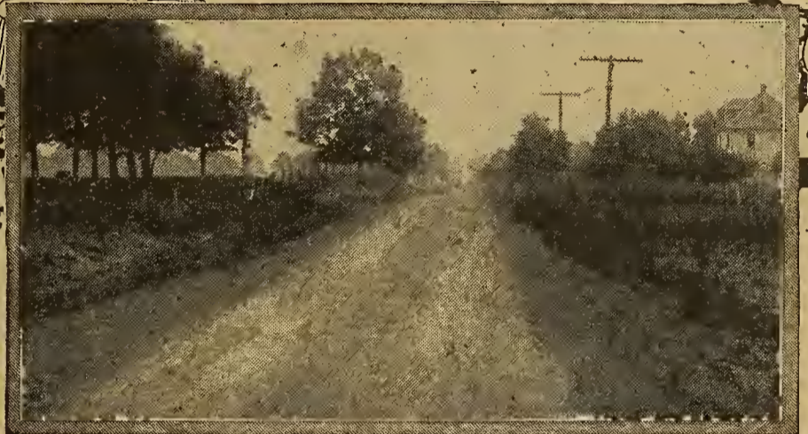
The same road showing what the use of "Tarvia-X" has done. Note smooth, dustless surface.
