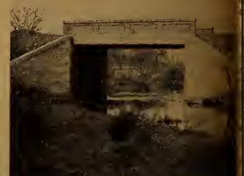
Nowadays concrete takes the place of the wooden bridge
