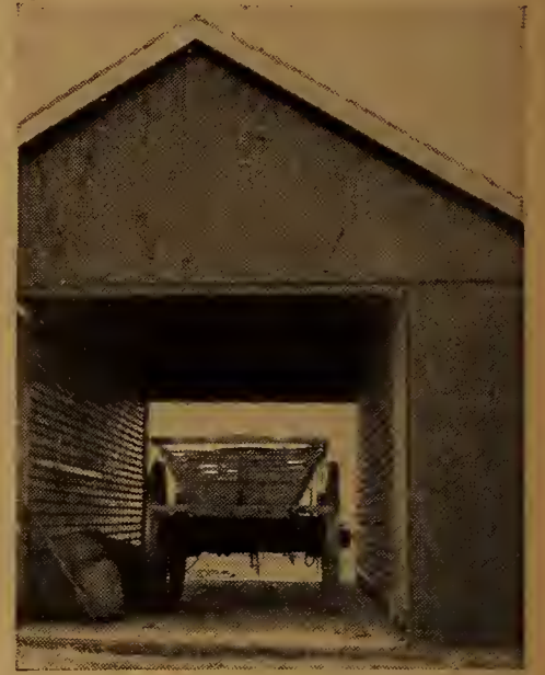
A lining of wire mesh keeps the rats out of this crib
