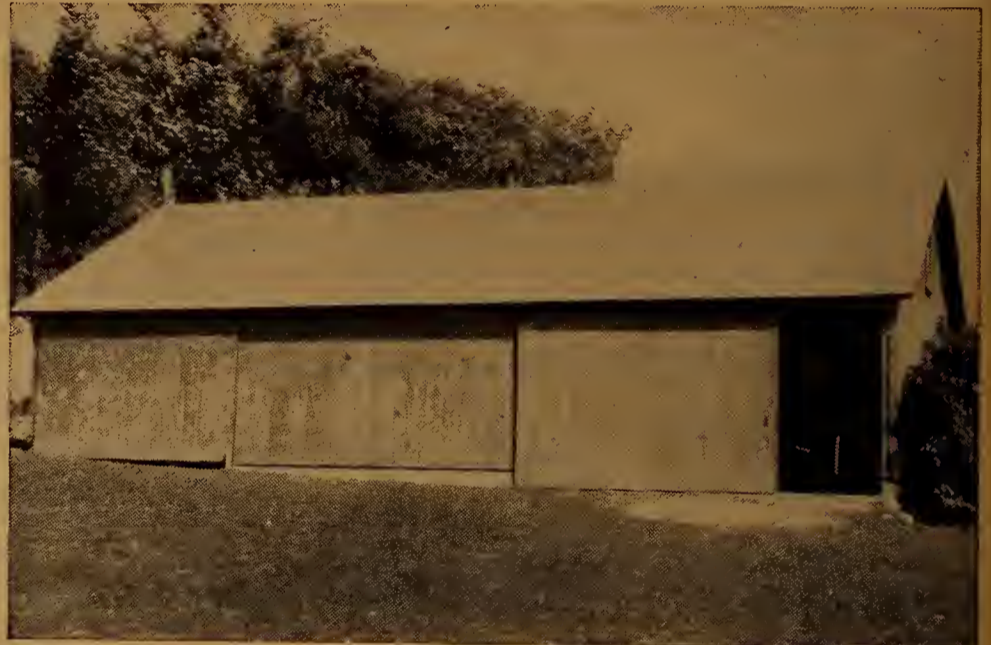
The openings in an implement shed must be large enough to accommodate the widest farm machinery
