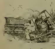
LIFTING HERSELF INTO THE DITCH.
