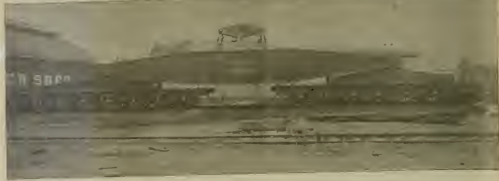
THE CAR HERE CARRIES THE KIEFF GEN TO CHICAGO. WEIGHT OF CAR AND LOAD, 445,000 POUNDS.
