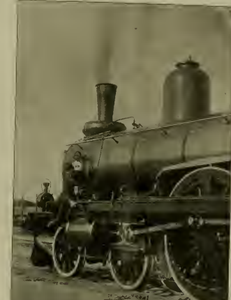
TAKING INDICATOR DIAGRAMS ON A SWEDISH LOCOMOTIVE.
