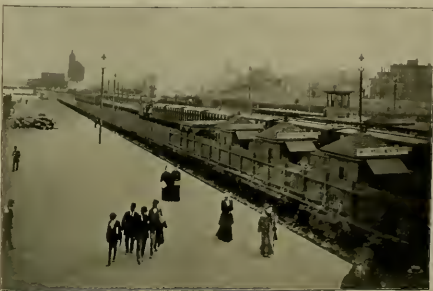
NO. 6. UNLOADING TRAIN CLEARED IN 55 SECONDS AFTER DEAD STOP. PLATFORM CLEARED IN 30 SECONDS AFTER DEAD STOP.
