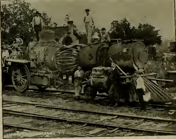
A STRANGE BOILER EXPLOSION.—AFTER WRECK WAS PICKED UP.
