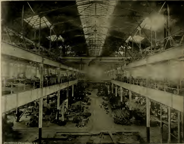
INTERIOR OF NEW SHOP—OLD SHOP ENTIRELY DESTROYED
