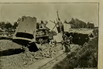
SHOWING ARRANGEMENT OF ROLLING STOCK AFTER FREIGHT TRAIN HIT COAL TRAIN.
