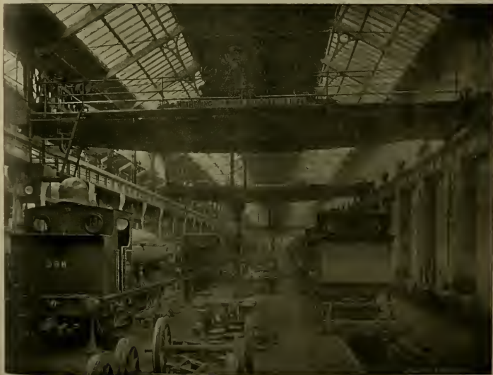
ERECTING SHOP LANCASHIRE & YORKSHIRE RAILROAD, HORWICH, ENGLAND.
