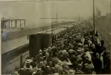
NO. 1. LOADING. DEAD STOP (LOOKING SOUTH)
