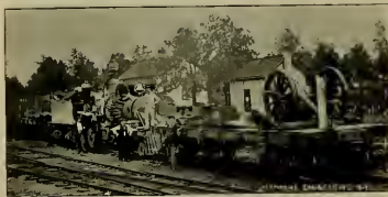
A STRANGE BOILER EXPLOSION.—READY TO BE TOWED HOME.
