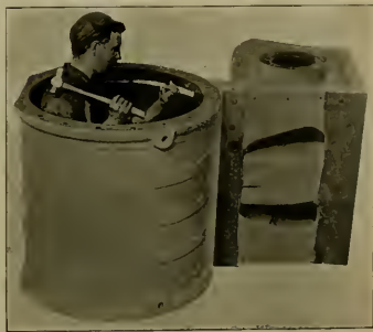
WORK ON THE CYLINDER OF SUBSEQUENTLY CONSTRUCTED LOCOMOTIVE.
