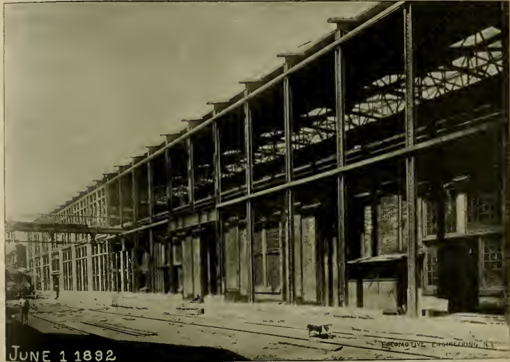
SHOWING NEW STRUCTURE OUTSIDE OF OLD SHOP.
