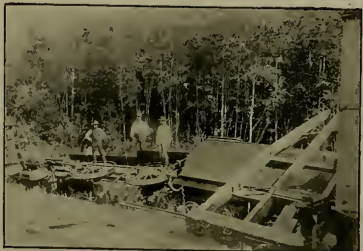
EARTHQUAKE WRECK AT PATRI, S. C., 120 MILES NORTH OF CHARLESTON, AUGUST 31, 1886.—FIREMAN KILLED.
