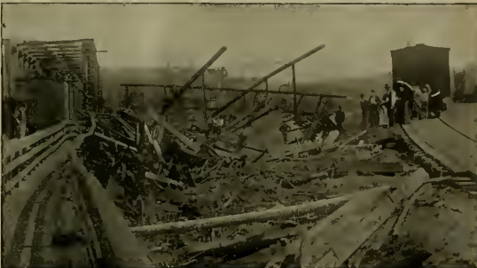
DESTRUCTION OF ILLINOIS CENTRAL BRIDGE, AT GALENA, ILL.
