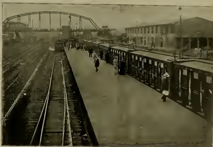
NO. 4. LOADING TRAIN FILLED IN 15 SECONDS AFTER DEAD STOP.
