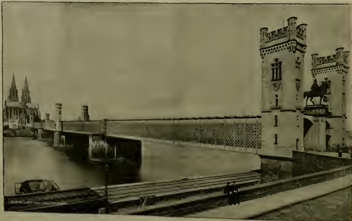
RAILWAY BRIDGE AT COLONE.
