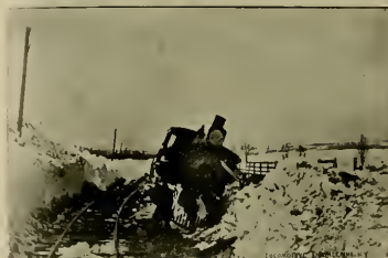
FORSAKEN—TRACK BUILT AROUND WRECK.
