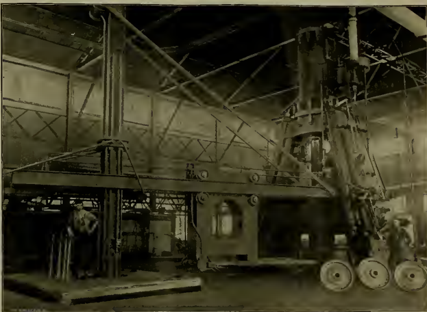
STEAM HAMMER IN BOIES' STEEL WHEEL WORKS, SCRANTON, PA.
