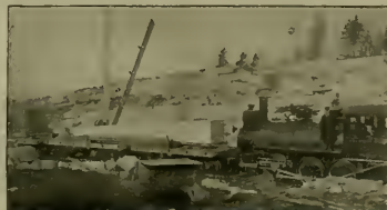
SIXTY-FOOT GRANITE SHAFT ON TWO CARS.
