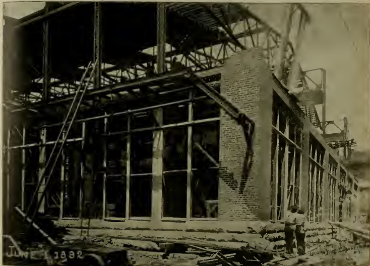
END VIEW, SHOWING PROGRESS OF THE WORK.
