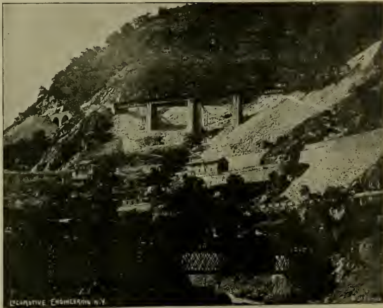
SOUTH SIDE OF ST. GOTHARD, LOOKING UP.
