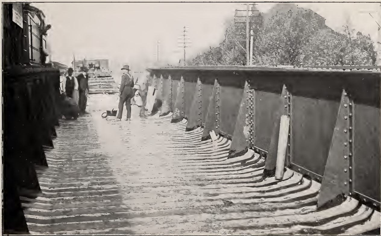
CHICAGO AND WESTERN INDIANA R. R. BRIDGES, CHICAGO, ILL., SHOWING APPLICATION OF HYDREX PER OUR NEW METHOD
