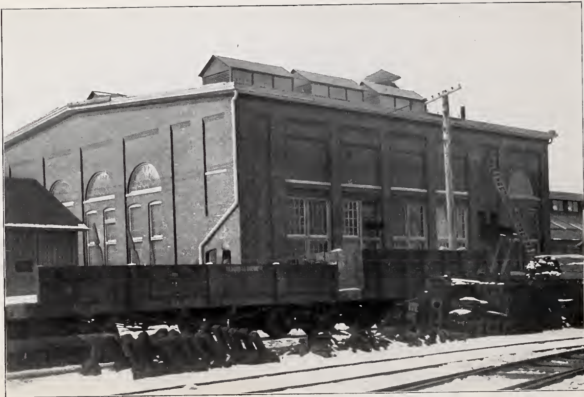
POWER HOUSE OF D. & H. R. R., BINGHAMTON, N. Y. FOUNDATIONS WATERPROOFED WITH HYDREX
