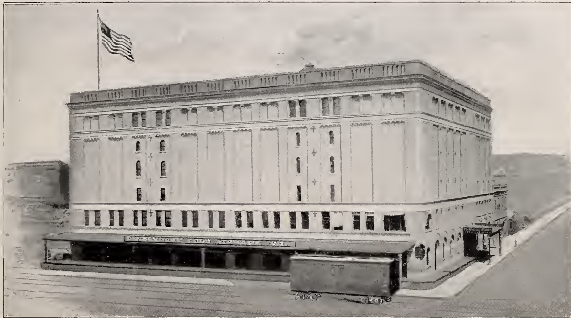
GANSEVOORT COLD STORAGE CO'S BUILDING, NEW YORK CITY. FLOORS WATERPROOFED WITH HYDREX
