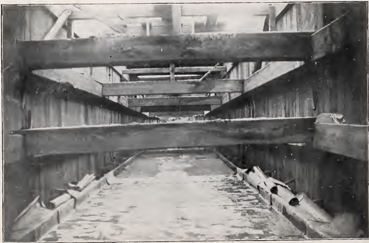
HYDREX BEING APPLIED IN TUNNEL WORK
