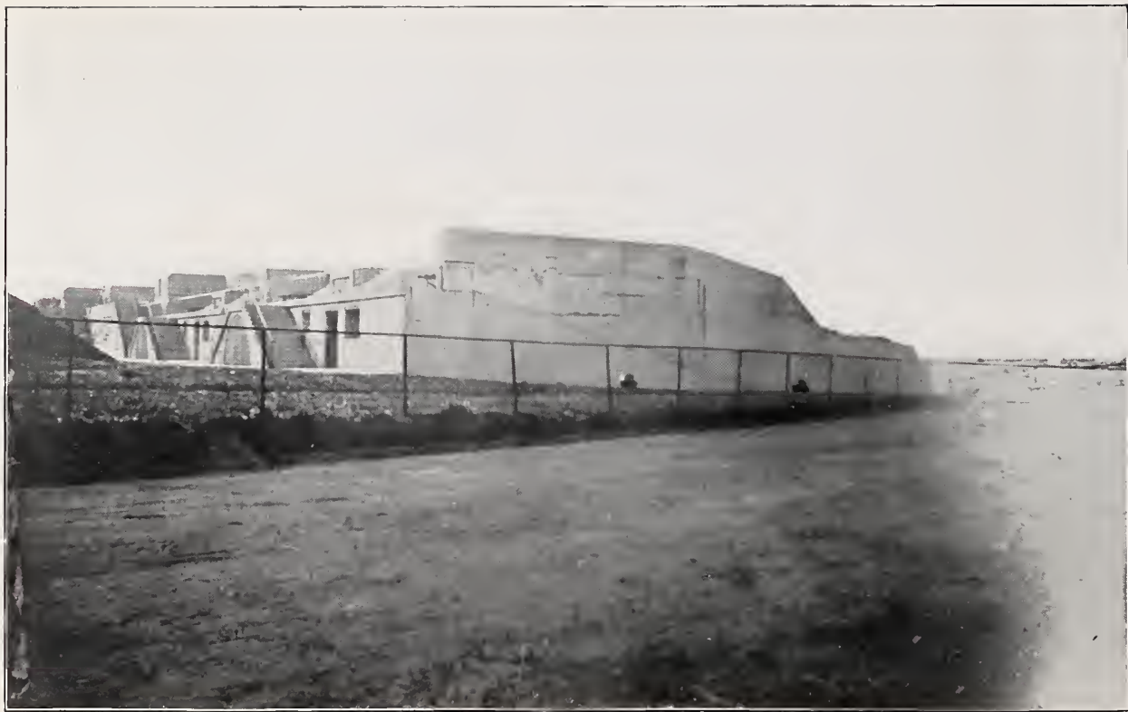
GOVERNMENT FORTIFICATIONS, FORT HAMILTON, N. Y. HYDREX LARGELY USED FOR WATERPROOFING MAGAZINES. 60,000 SQUARE FEET USED IN THIS BATTERY
