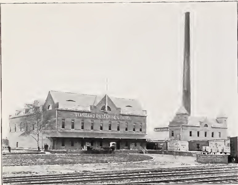
STANDARD BUTTERINE CO.'S BUILDINGS, WASHINGTON, D. C. THREE LAYERS USED TO WATERPROOF FLOORS
