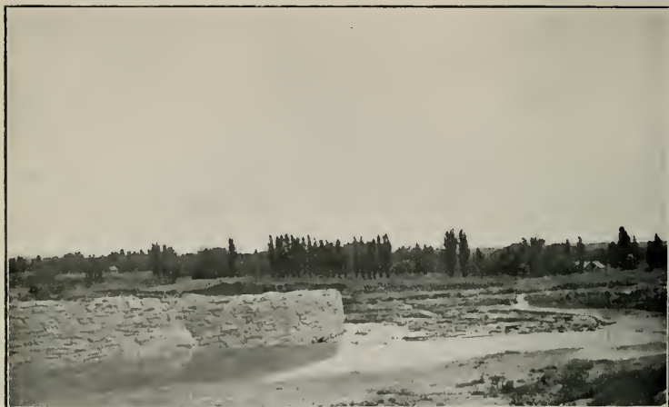
WOODRUFF DAM, AFTER ONE OF THE FREQUENT WASHOUTS
