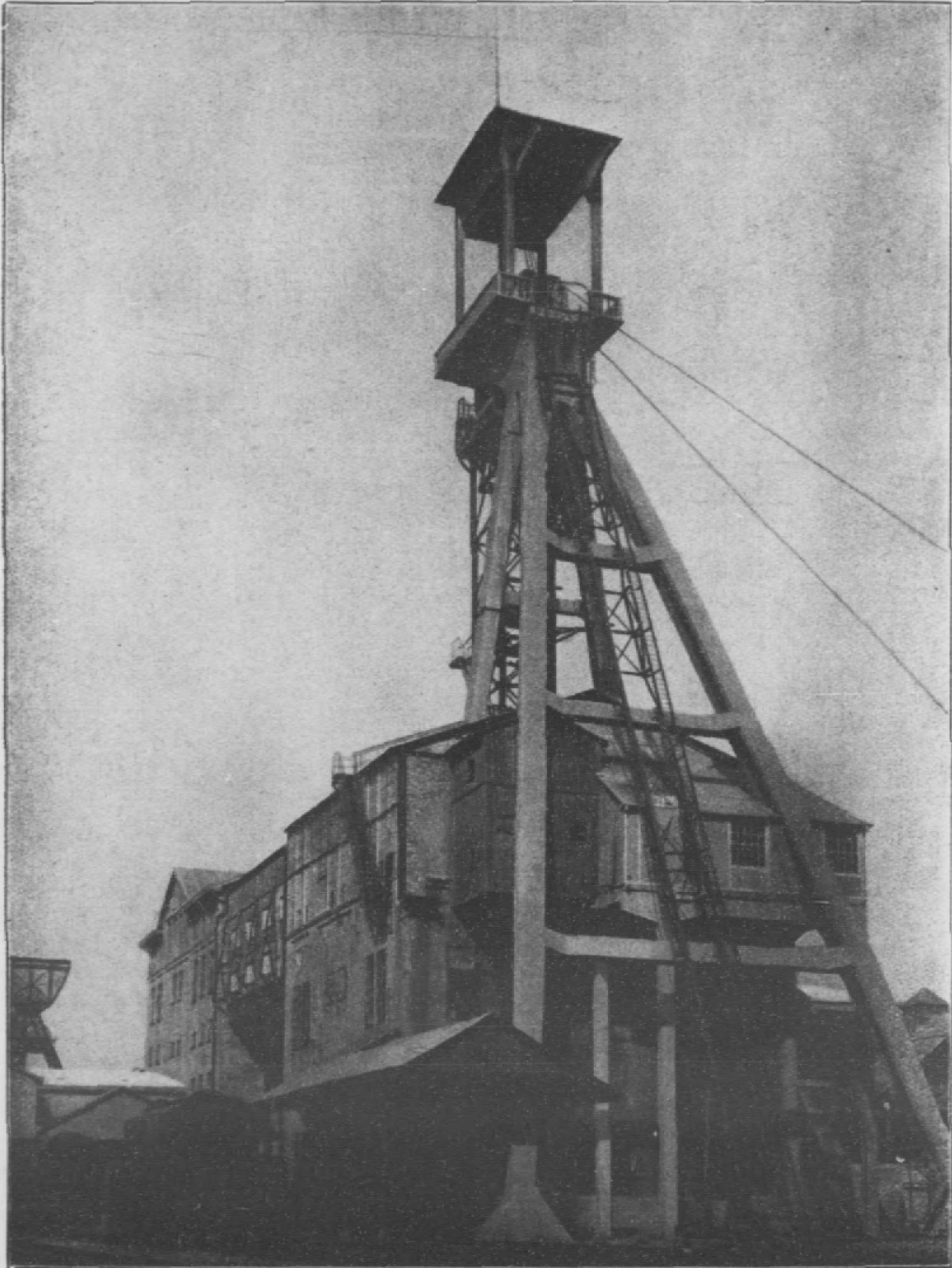
Exterior view of Potash mine Showing concrete pit-head.
