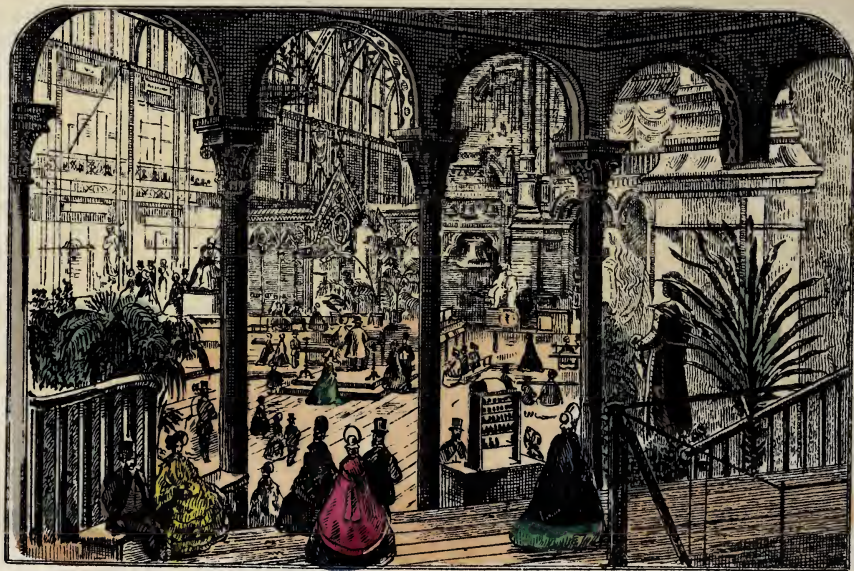
Western Dome, from entrance to Staircase.
