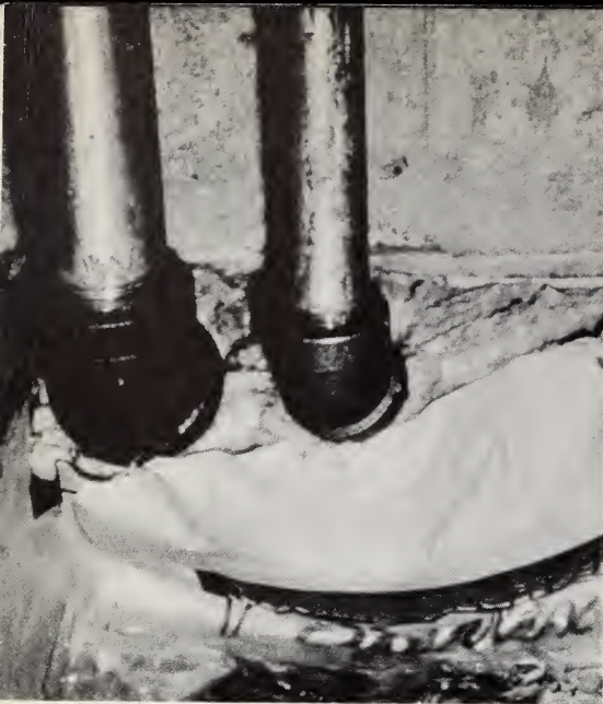
Fireproof insulation is applied carefully around piping.
