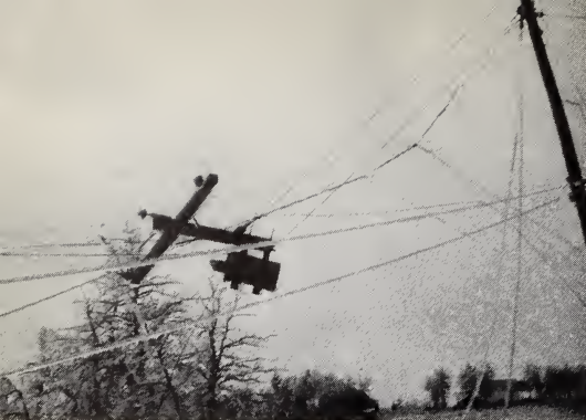
Broken poles could be seen everywhere in northern Alabama.
