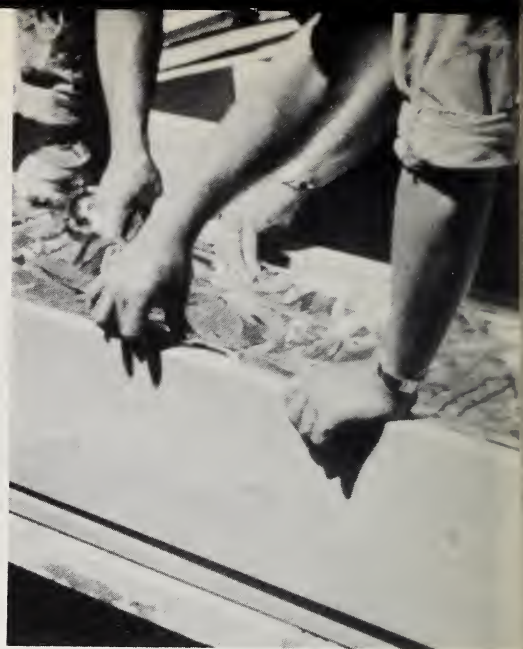
Visitors saw how insulation must be carefully installed.
