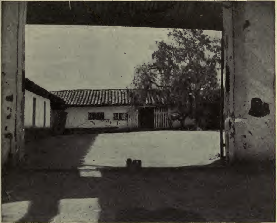
THE STABLE PATIO
