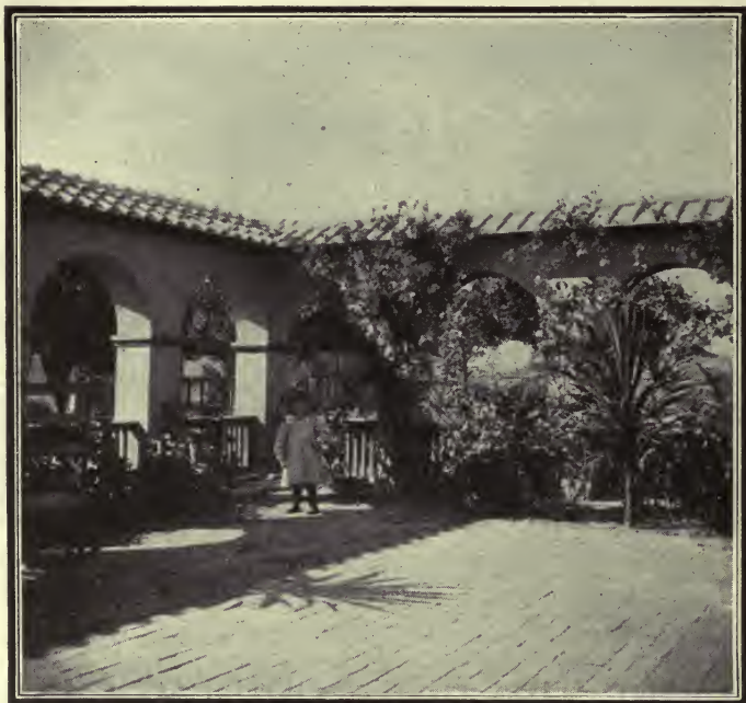
INTERIOR OF PATIO
