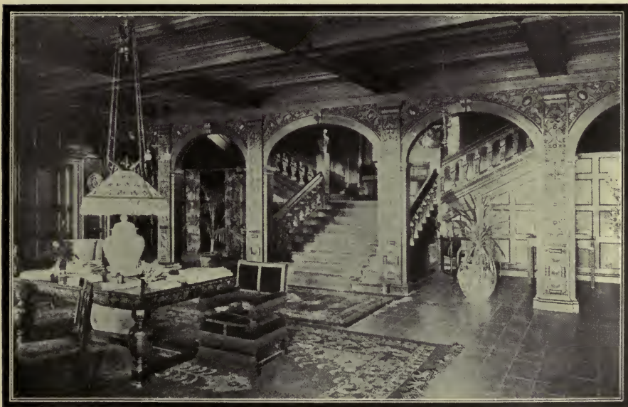
THE STAIRCASE HALL
