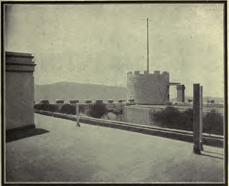
ON THE ROOF
