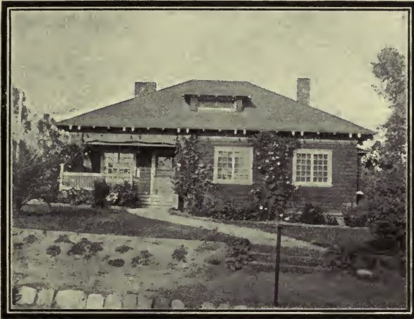
THE APPROACH TO THE SQUARE COTTAGE
