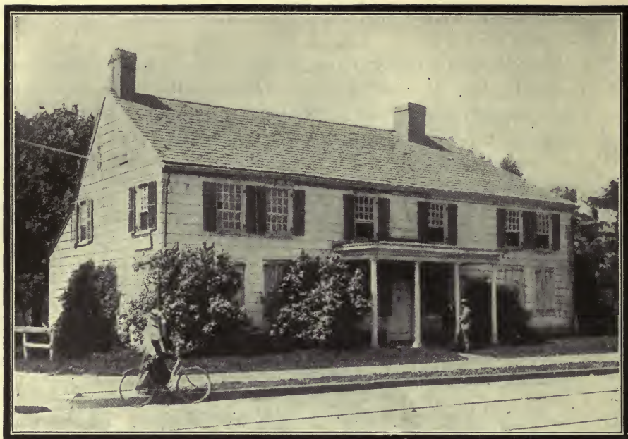
THE BERGEN HOMESTEAD, THE OLDEST HOUSE IN FLATBUSH
