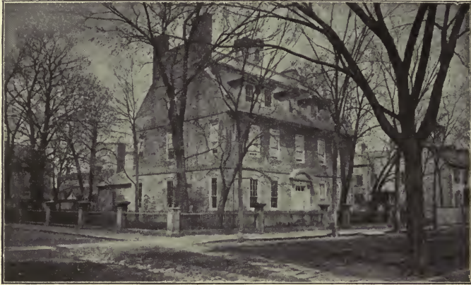
THE WARNER HOUSE, PORTSMOUTH, N. H., BUILT BY CAPTAIN McPHÆDRIS IN 1723
