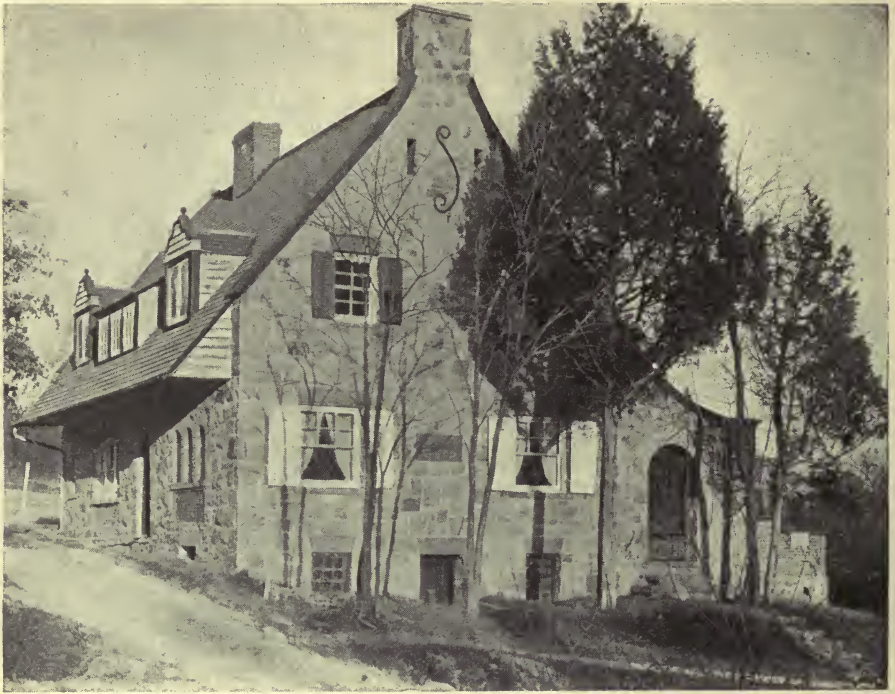
PRINCESSGATE—GABLE AND DORMERS
