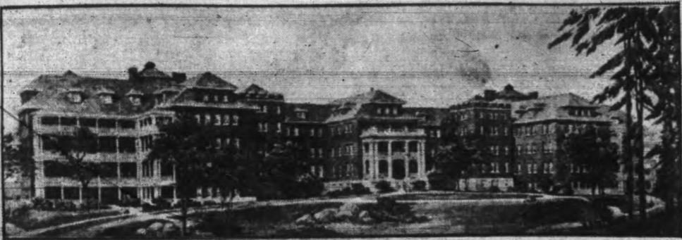
NEW PROVINCIAL HOSPITAL FOR INSANE BEING BUILT AT COQUITLAM
