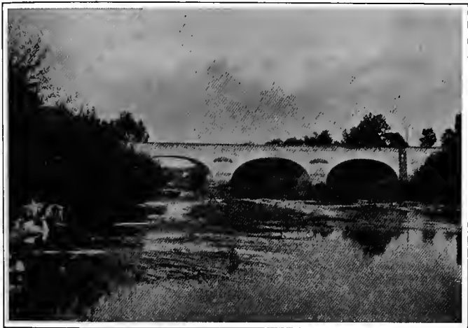
Bridge at Berry-au-Bac.
