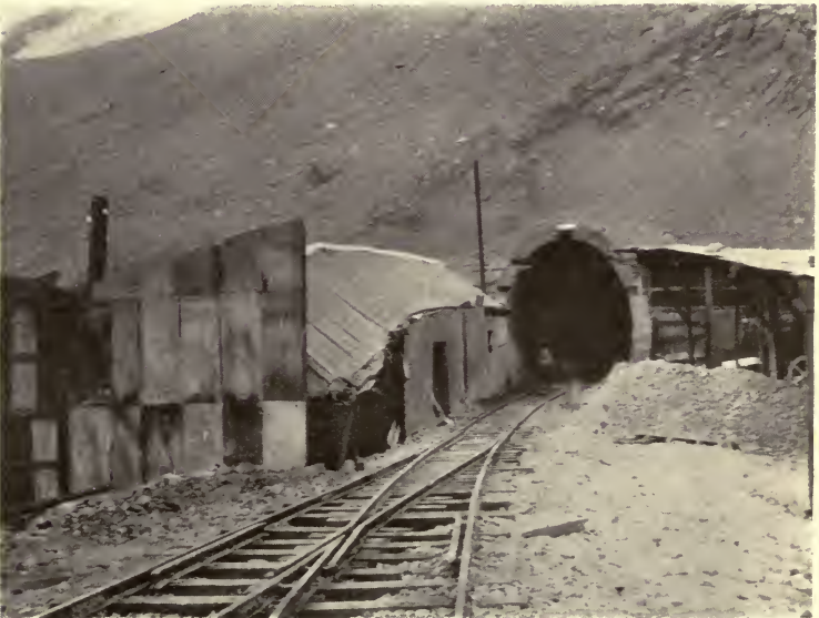
ENTRANCE TO THE SUMMIT TUNNEL THROUGH THE ANDES. (CHILEAN SIDE)
