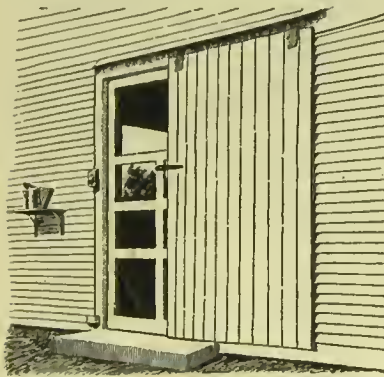
FIG. 18. — Honey-house door. The wooden door rolls clear of the opening and the screen door swings both ways.
