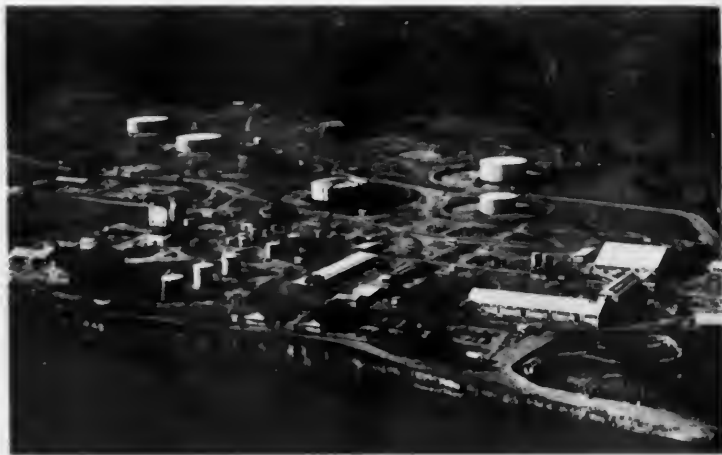
OIL TANKS OF THE TROPICAL OIL COMPANY AT BARRANCA BERMEJA
