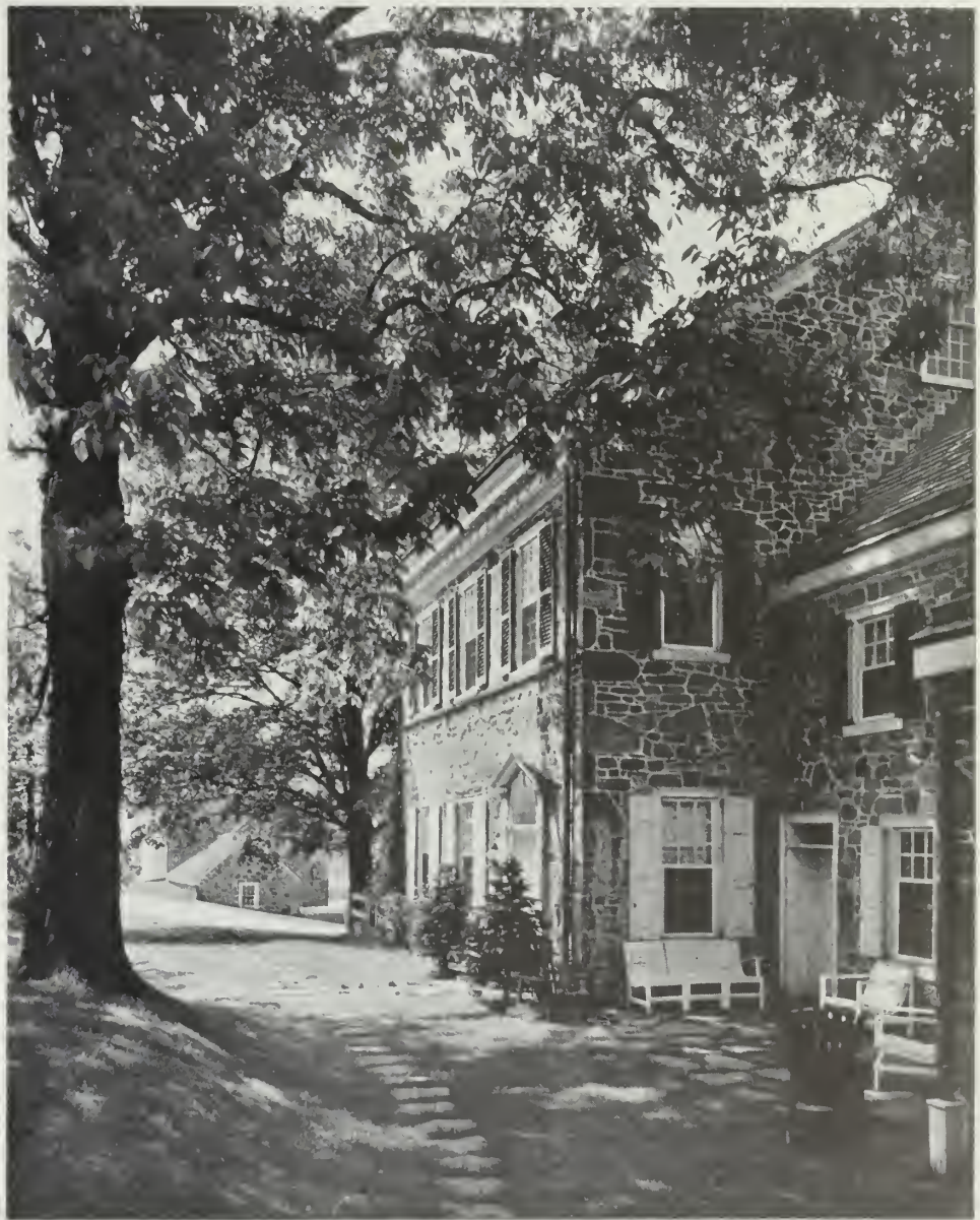
The entrance front of this fine old Colonial iron-master's house faces toward the southwest
