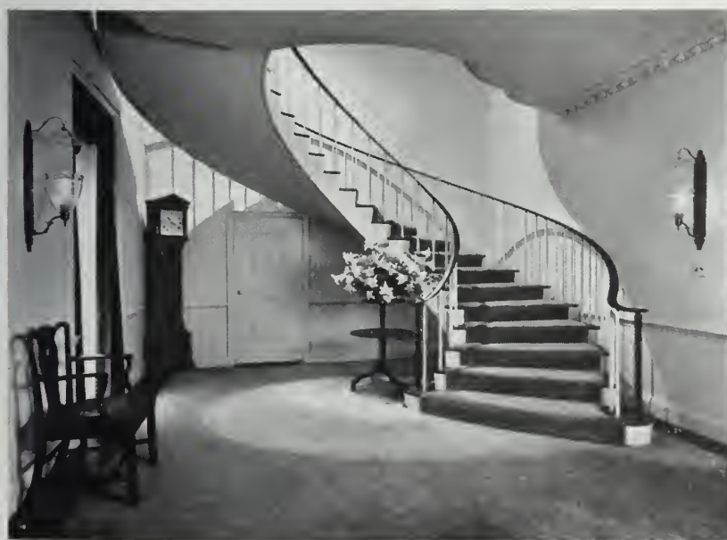
The main staircase at end of entrance hall is a true ellipse in plan
