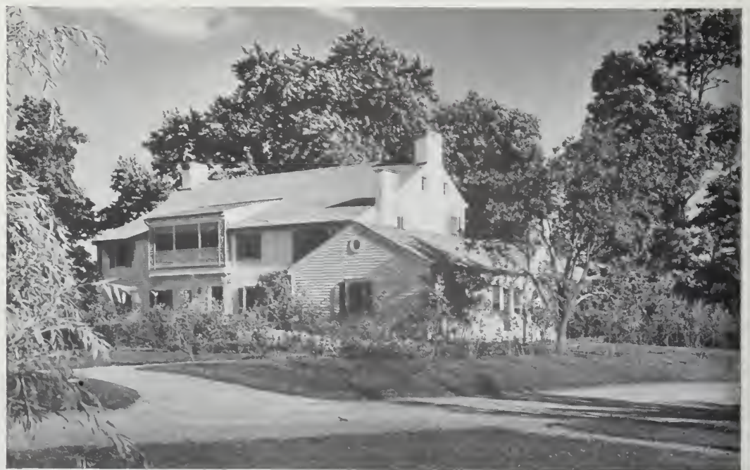
The house was completed in 1812 by an Indian trader whose taste and skill were impeccable
