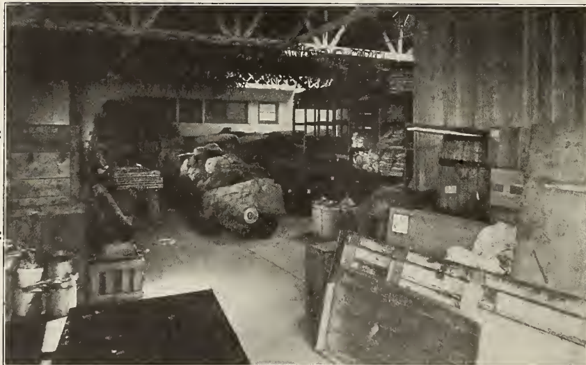
A section of the vast supply room of the newly completed Anderson Boarding and Supply home in Hollywood where is stored equipment that would supply an army comfortably.
