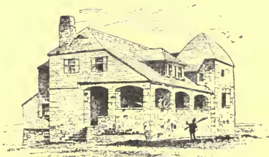
COTTAGE AT JAFFREY POINT.
