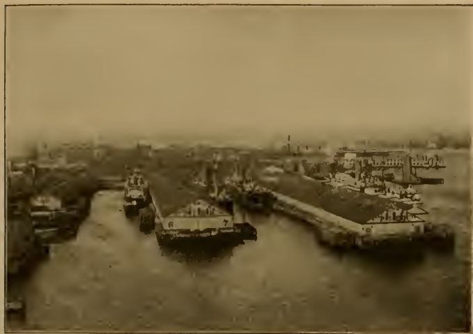
RAILROAD PIERS IN BALTIMORE HARBOR.
