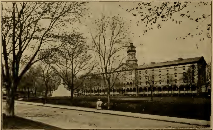
BUILDING OF THE NAVAL ACADEMY, ANNAPOLIS.
