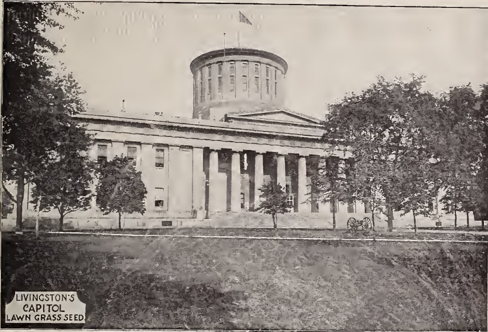
The illustration herewith shows a small portion of the beautiful grounds surrounding the Capitol of the State of Ohio. One of the most attractive features of these grounds are the splendid lawns—made from
