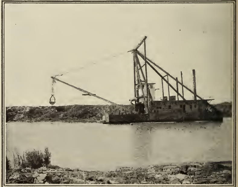
THE DREDGE, "GOLDEN GATE," BUILDING A LEVEE ON THE DELTA LANDS, SAN JOAQUIN VALLEY, CALIFORNIA.
