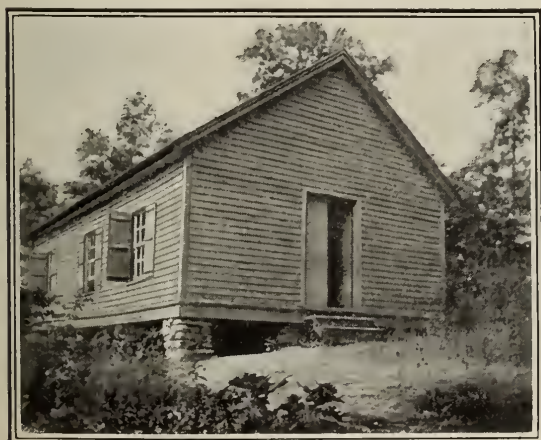
The old building.
