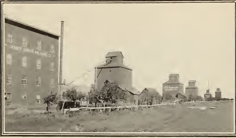
GRAIN ELEVATORS AT HARTNEY, MANITOBA.
