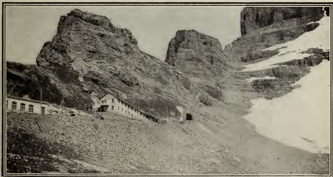
THE GLACIER STATION AND THE EIGER TUNNEL.
