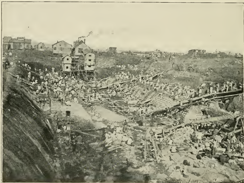
Constructing a Dry Dock at Dalny
