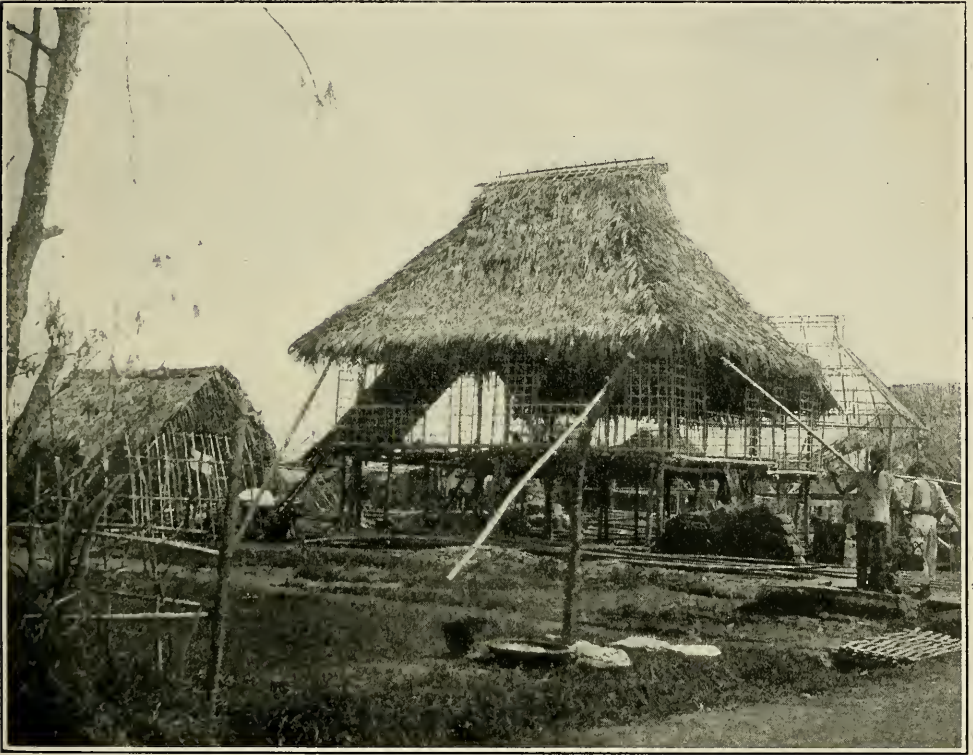
Nipa House Under Construction
