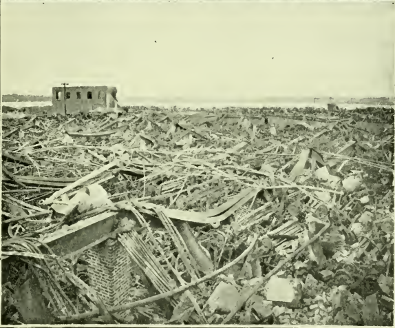
NO. 6 WEAVESHED AT THE NAUMKEAG MILLS BEFORE AND AFTER THE FIRE Photographs by M. E. Robb, Salem
