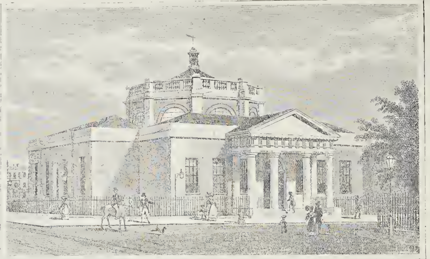
The Westminster Guildhall or Sessions-House, now in course of Demolition.
