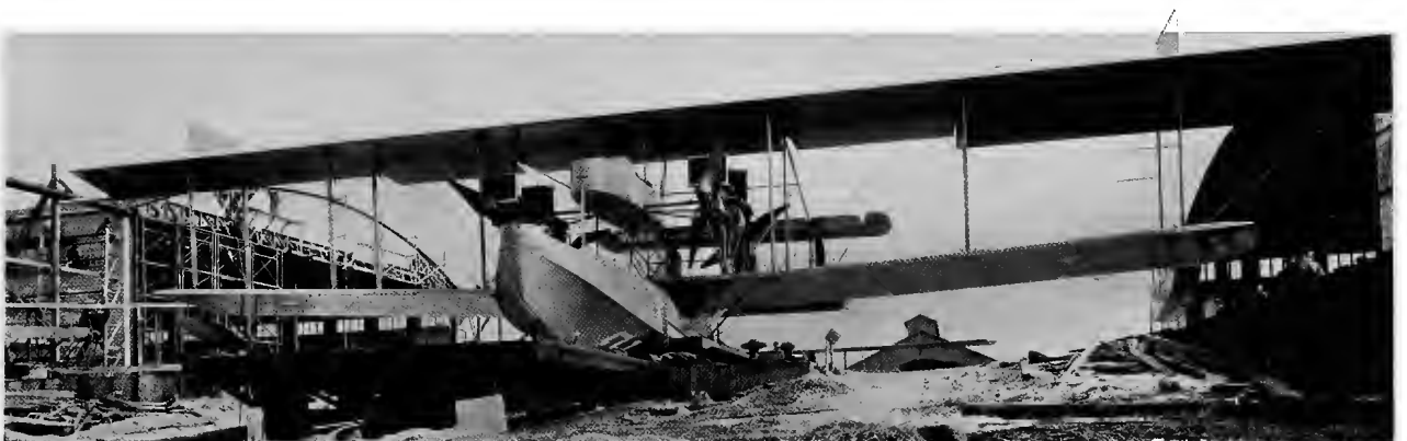
The NC-2 on the marine railway at Rockaway
