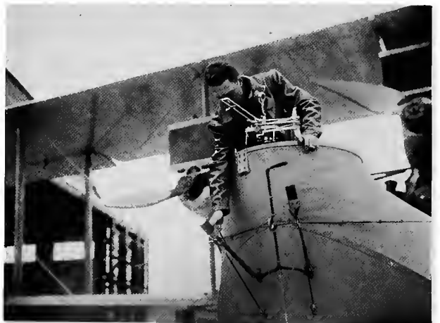
Photo, Edwin Levick, N. Y. The "Drift-Indicator" above and "Landing Flares" below Bow of one of the NC's
