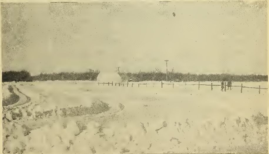
Figure 12. - A series of snow traps. The snow cloud in the center of the picture is caused by a rotary plow engaged in widening work.
