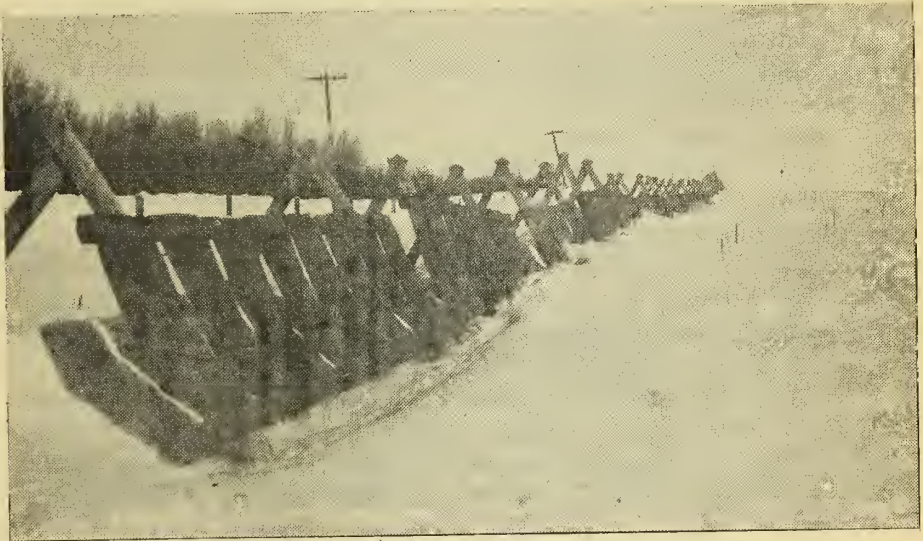
Figure 11. - A snow fence made from discarded bags and framed guard-rail timber.
