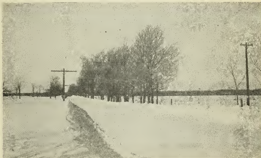
Figure 5. - An open road, in the State of Michigan, where the cleared way has been widened with truck-plow attachment.
