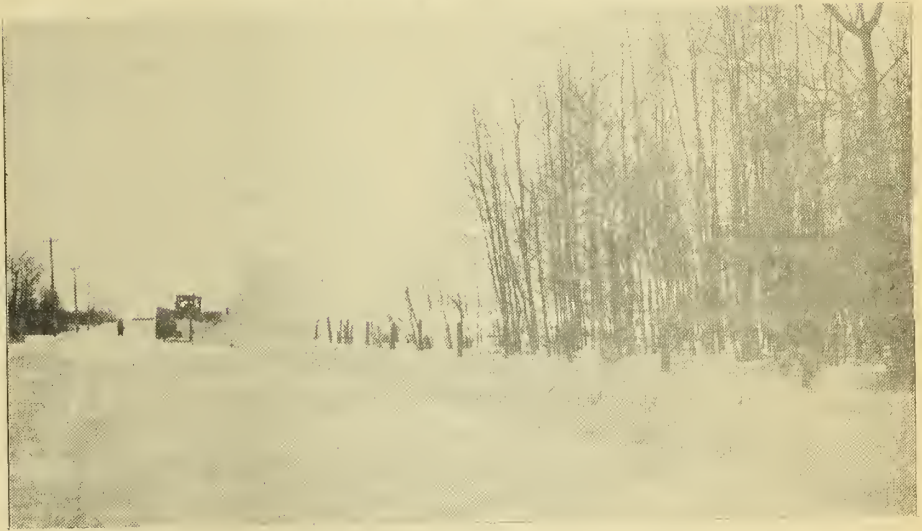
Figure 8. - A rotary plow in action, widening a cut.
