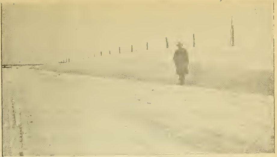
Figure 7. - A vertical snow bank with level top. This cut was widened with a rotary plow.
