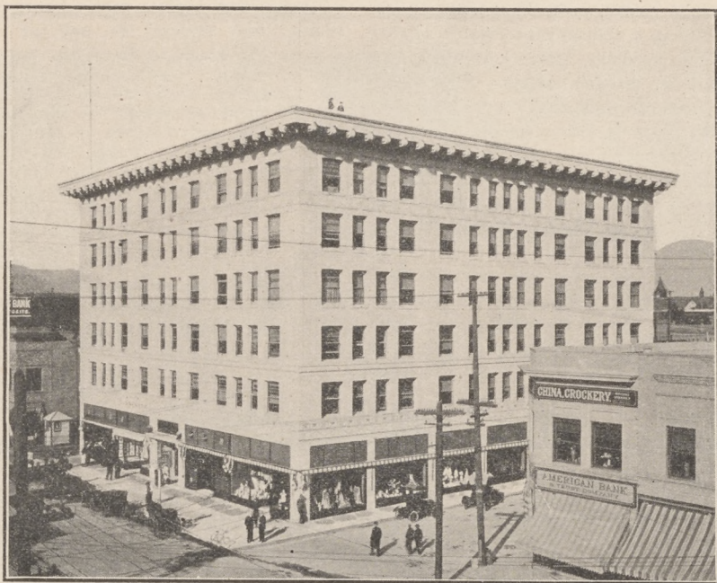
Chamber of Commerce Building
