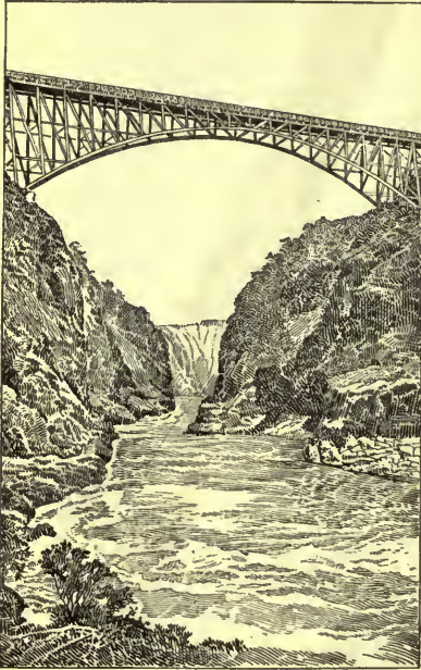
BRIDGE ACROSS THE ZAMBESI RIVER, NEAR VICTORIA FALLS
