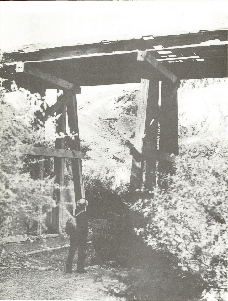
T & T TRESTLE OVER WILLOW CREEK
