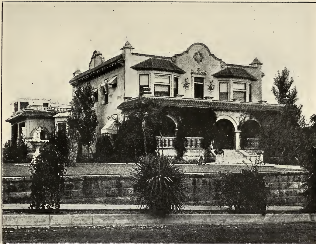
A TYPICAL FORT WORTH RESIDENCE Home of a Texas cattleman
