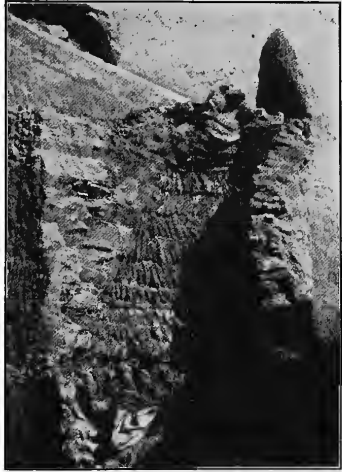
Section of a Pre-Sargonic Well. Bricks laid in Herring-bone Fashion
