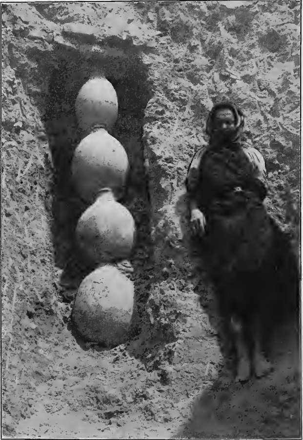
Perpendicular Drain composed of Jars. About 200 B. C.
