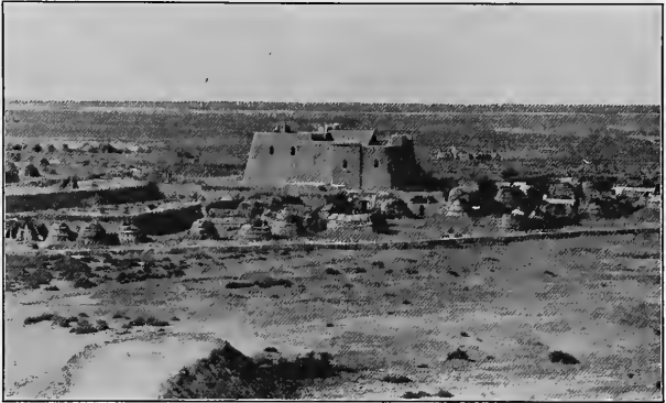
Headquarters of the University of Pennsylvania's Fourth Expedition at Nuffar Mefîl surrounded by gardens and reed-huts at the south foot of the ruins. The 'Afej swamps in the background.
