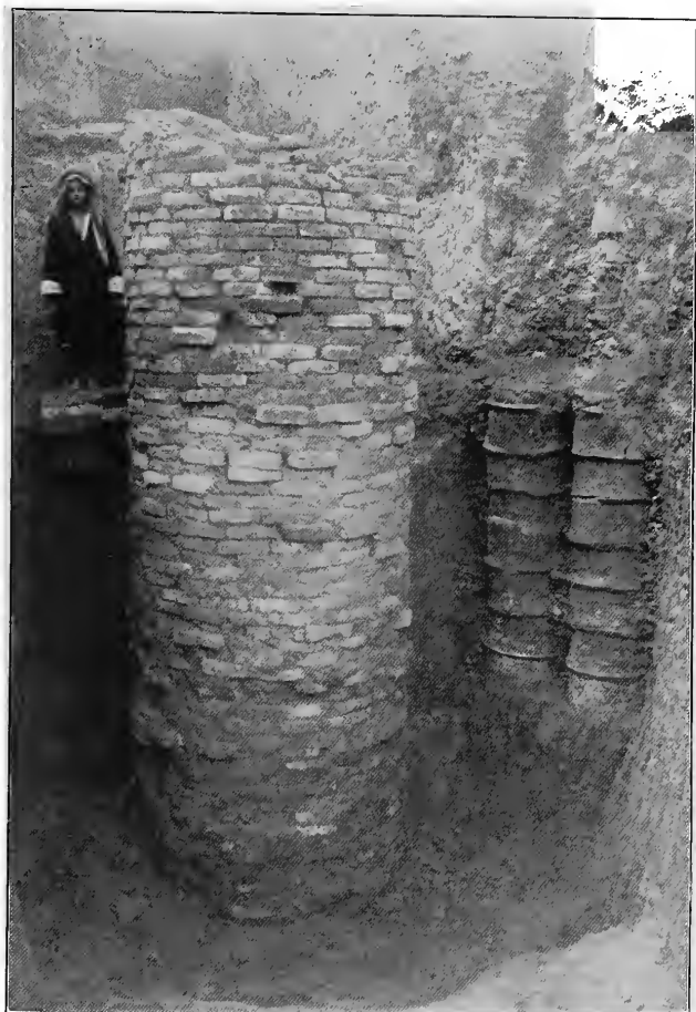
Well built of Bricks and Two Terra-Cotta Drains
