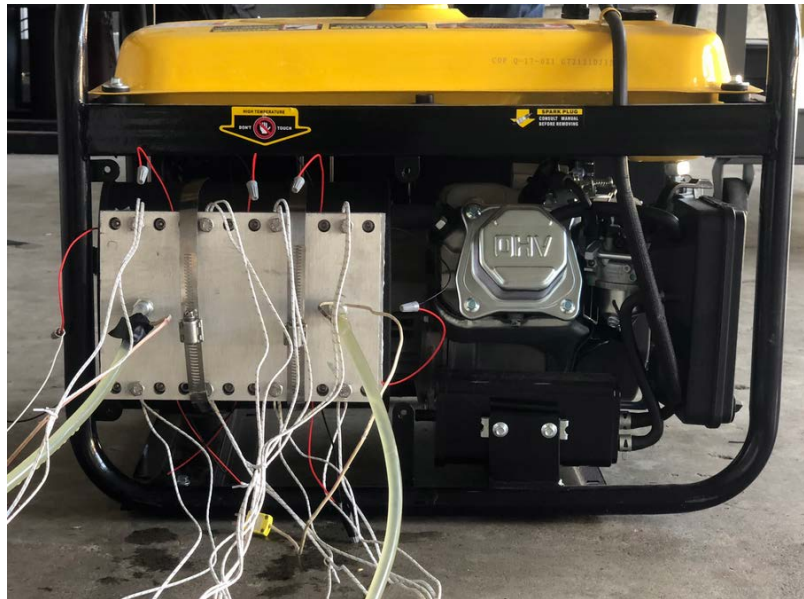
Figure 15. Thermoelectric Generator Waste Heat Harvesting Prototype Mounted to Muffler of Generator
