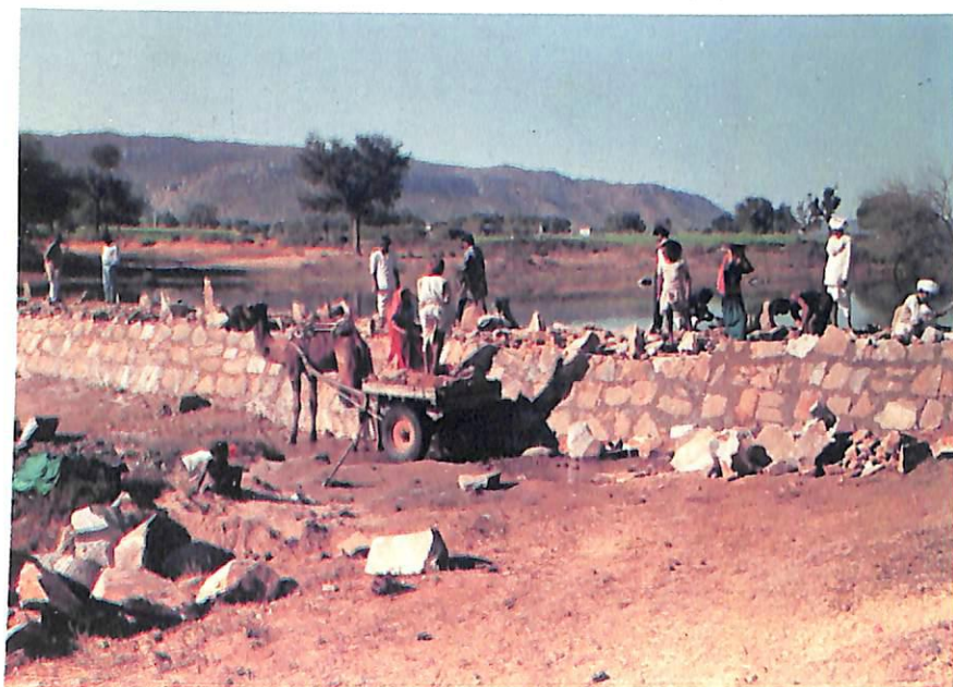
Jabbar Sagar Dam during construction (Hamirpur)
