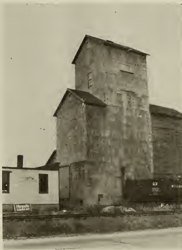
HAMEL CO-OPERATIVE GRAIN COMPANY'S ELEVATOR, WORDEN, ILL.
