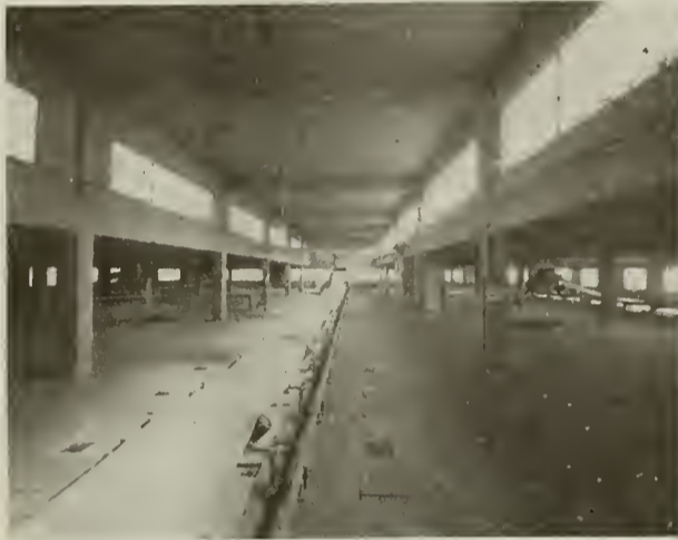
VIEW OF CONVEYOR GALLERY OF THE MURRAY ELEVATOR
