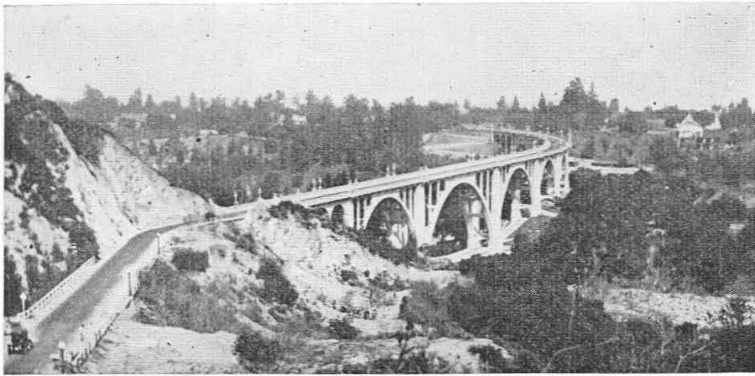
COLORADO STREET BRIDGE
