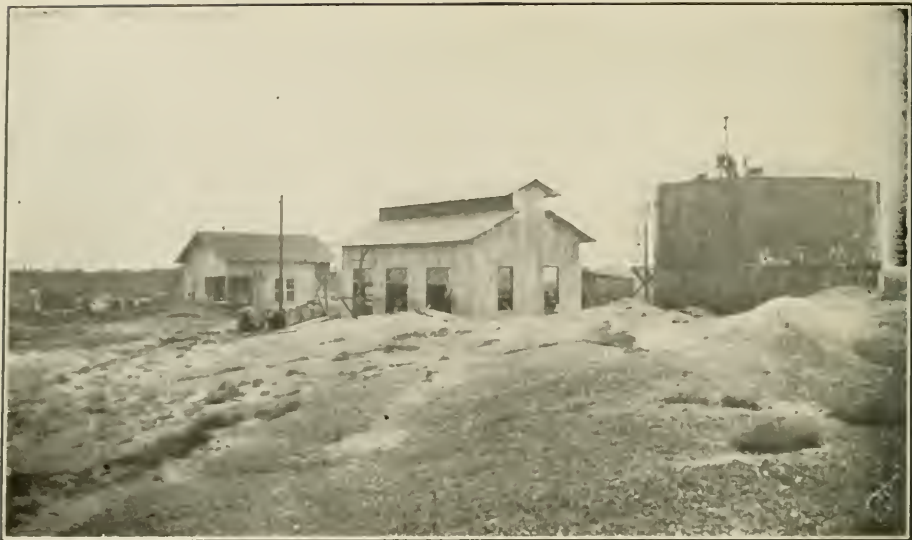
Storage Plant in Construction at Isabella de Sagua, Texas Co.
