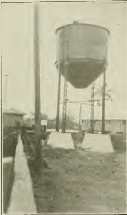
Oil Tank of Sinclair Oil Company, Guines, Cuba.
