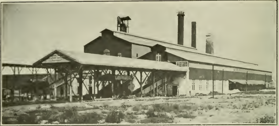
Central "Toledo"—General View
