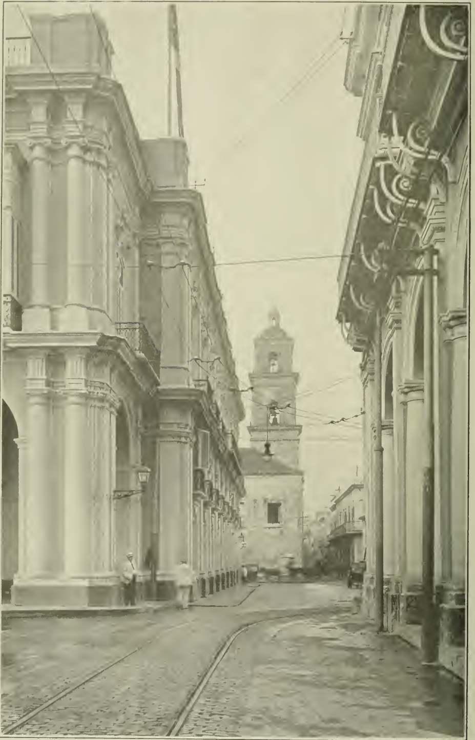
Old Sto. Domingo Church, Havana. (The Building on the Corner With the Steeple.) Just Opposite is the Old Presidential Palace.
