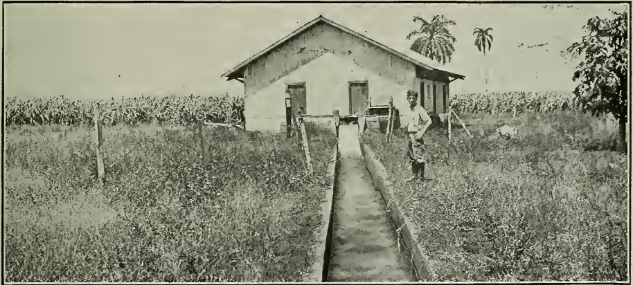
Cement Irrigation Canal and Pump House, SOCORRO.
