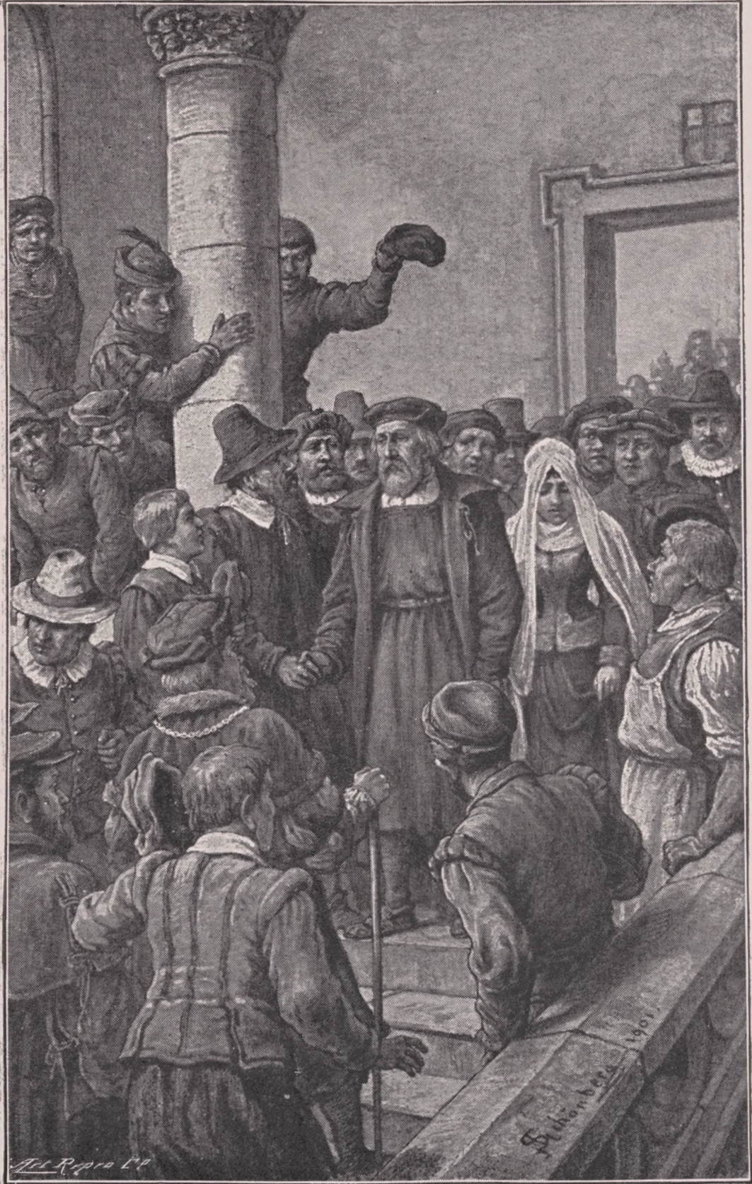
SOME CLUNG TO THE PILLARS, SOME GOT UP INTO THE WINDOWS.
