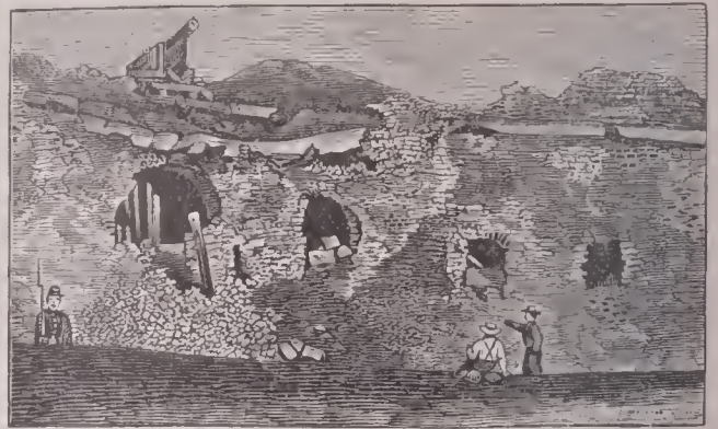
FIG. 4.—Fort Pulaski: front view of breach, from opposite side of ditch.
