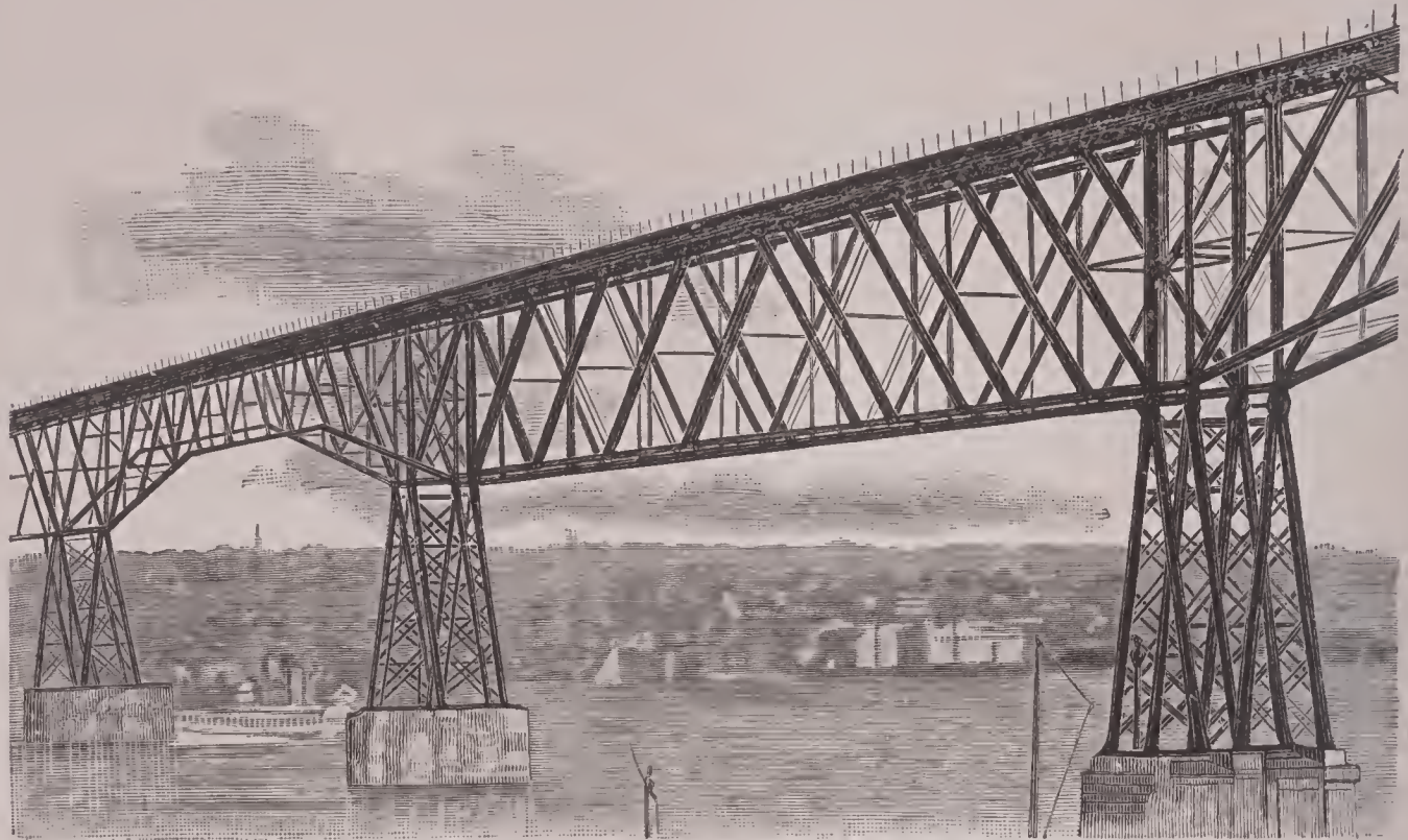
FIG. 27.—Poughkeepsie cantilever bridge, 1889.
