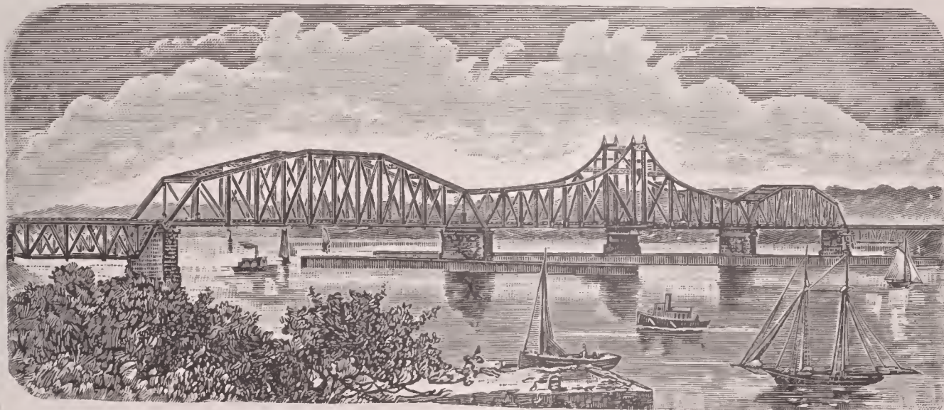
FIG. 25.—Thames river bridge, New London, Conn., 1890.
