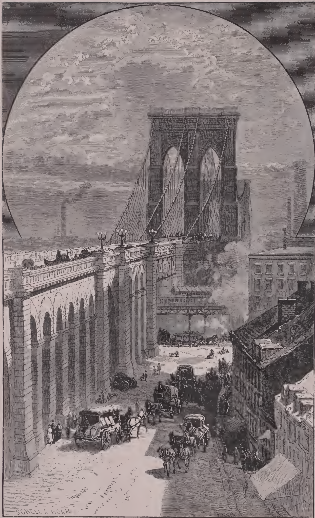
THE APPROACH TO THE EAST RIVER BRIDGE—(NEW YORK SIDE).
