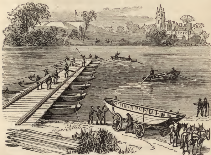
CONSTRUCTING A PONTOON-BRIDGE.
