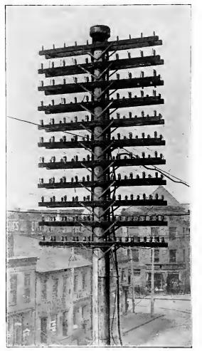
Fig. 325.—Pole Equipped with Cook Terminal.
