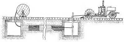
Fig. 339.--Drawing in by Steam Power.
