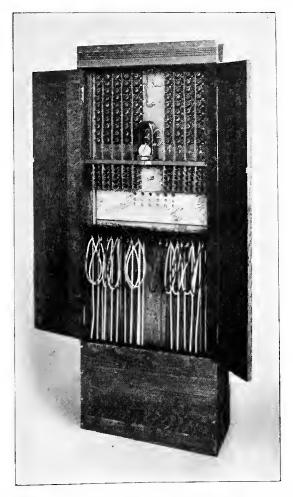
Fig. 170.-Sterling Electric Co.'s 100-Drop Switch-Board.
