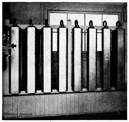
Fig. 327.—Interior Cable Heads.
