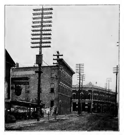
Fig. 326.—Cable Terminal Box with Balcony.
