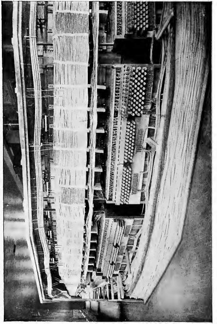
Fig. 212.--Rear View of Switch-Board, Showing Wiring.
