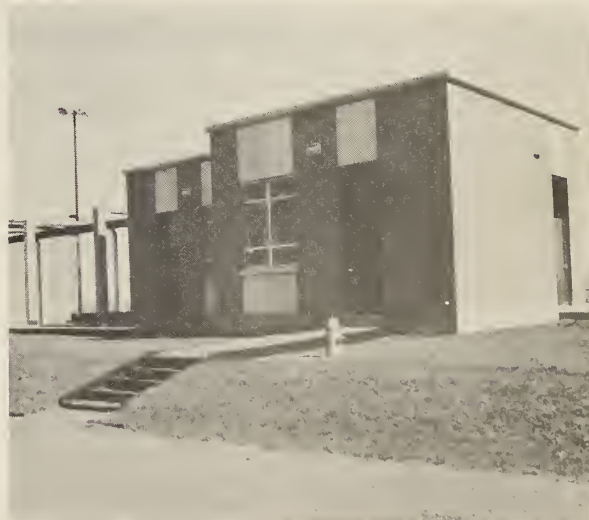
PLANT PUMPING STATION
