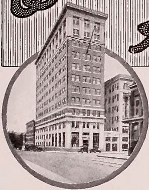
City National Bank Building, Shreveport, La. Architects, Languinet & Statts, Fort Worth, Texas; Associate Architect, E. F. Neild, Shreveport, La.; Gen'l Cont., Central Contracting Co., Houston, Texas; Roofers, H. H. Bain Sheet Metal Works, Shreveport, La.
