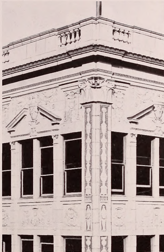
KRESGE STORE, BOSTON Newhall & Blevins, Architects Geo. A. Fuller Co., Builders Entirely of Atlantic Terra Cotta
