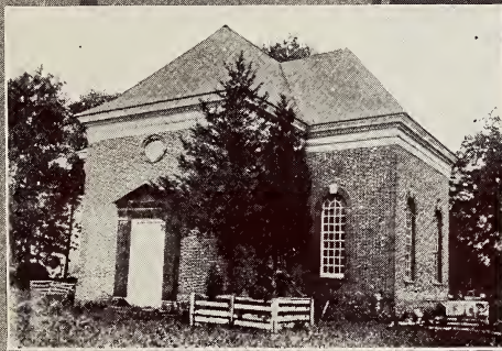
CHRIST CHURCH Showing remains of the old marble slabs over KING CARTER and his wives, JUDITH ARMISTEAD and BETTY LANDON.
