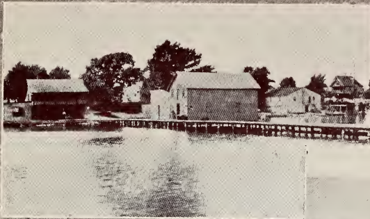
View of WEEMS' WHARF
