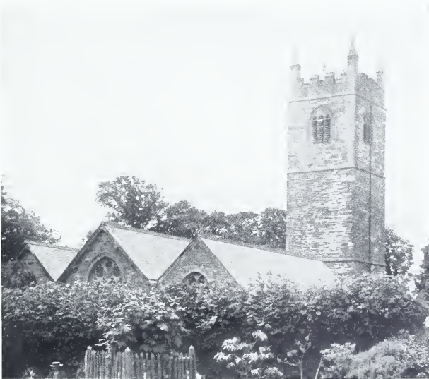
ST. TUDY CHURCH, CORNWALL, IN WHICH LOWER WAS BAPTIZED AND BURIED
