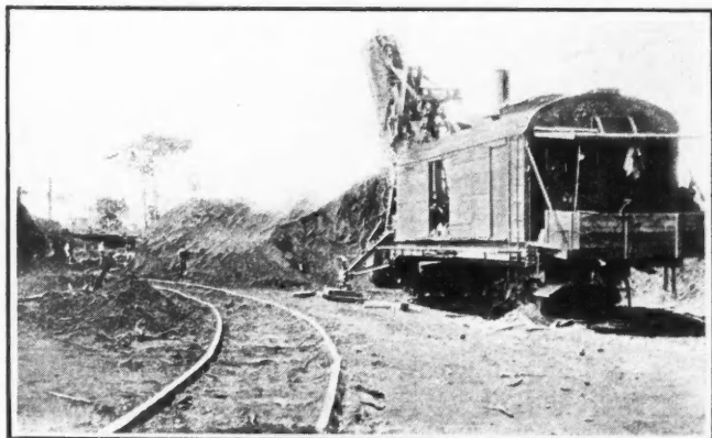
Excavating the site for the Bwana M'Kubwa plant
