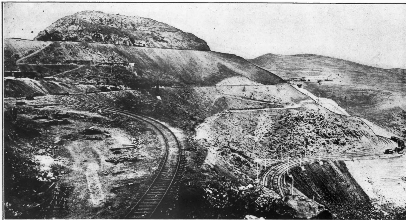
APPROACH TO STEAM-SHOVEL WORKINGS AT TOFO, COQUIMBO, CHILE
