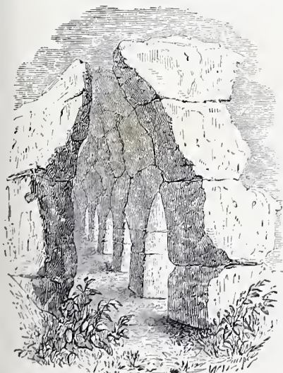
Fig. 10. PART OF THE WALLS OF TIRYNS.
