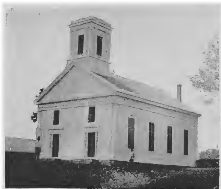
CONGREGATIONAL CHURCH (MONTVILLE CENTER).
