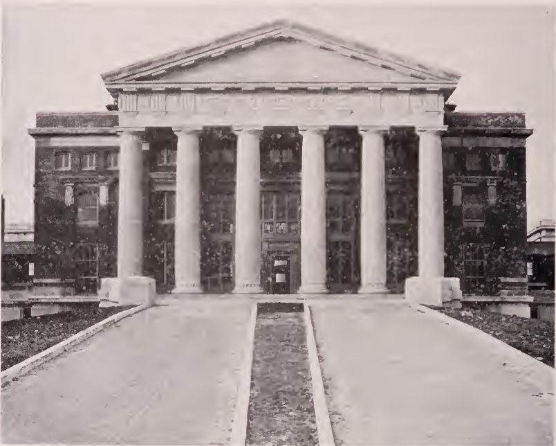
Main building of Peter Bent Brigham Hospital, Boston.
