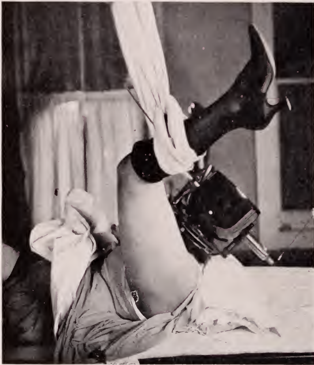
Fig. 1.—Close up side view, showing the method of supporting the legs and the x-ray tube in position.
