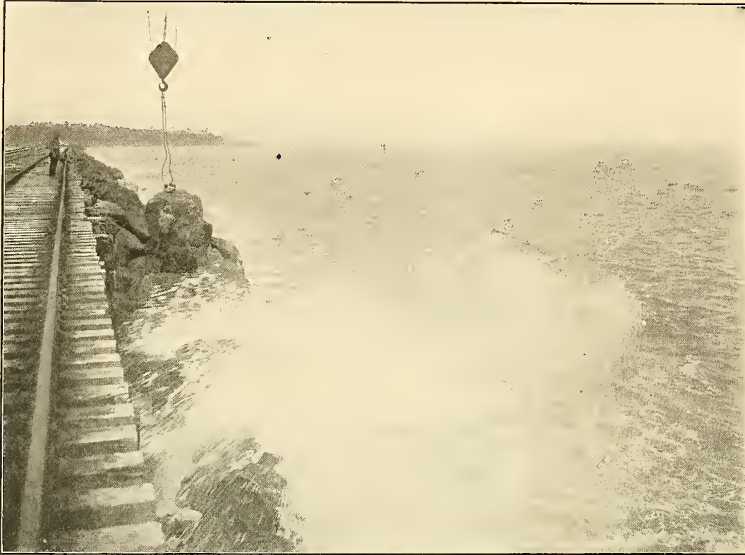
TORO POINT BREAKWATER
