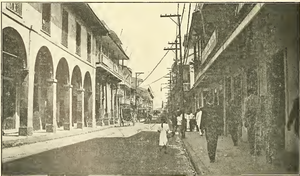
A STREET AFTER PAVING
