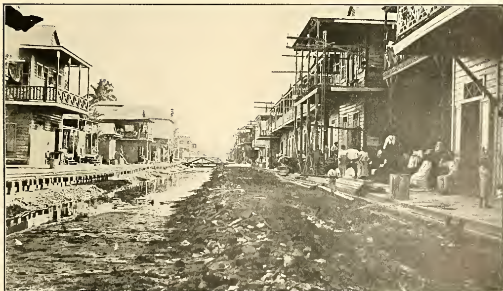
AN OPEN SEWER IN A COLON STREET
