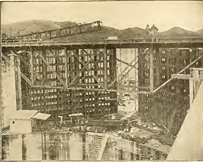
BUILDING AN UPPER TIER OF LOCKS
