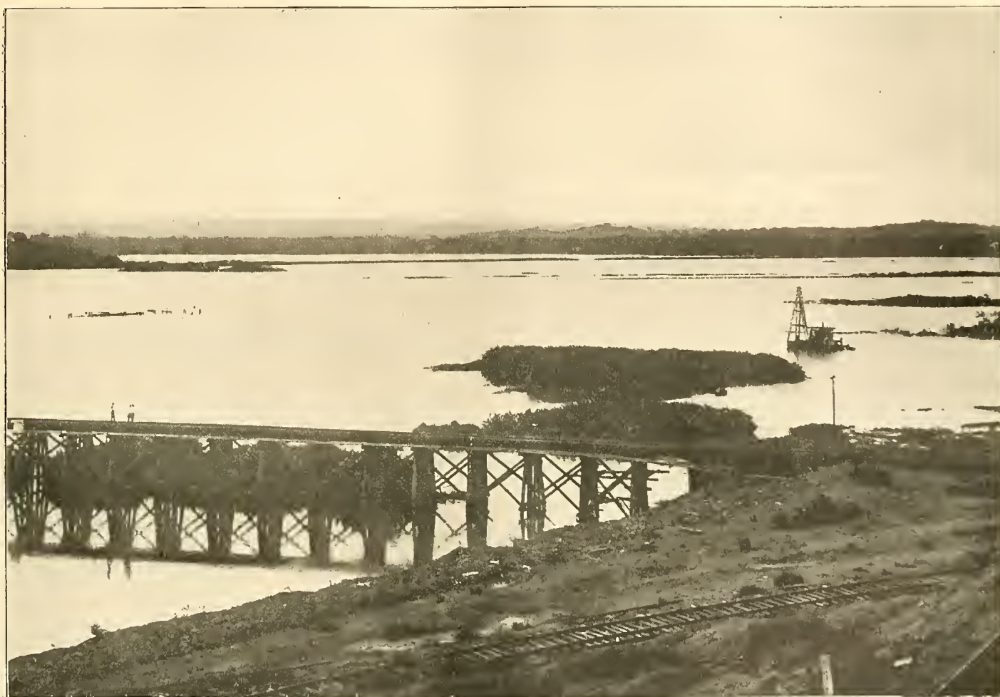
GATUN LAKE. FLOATING ISLANDS MASSED AGAINST TRESTLE
