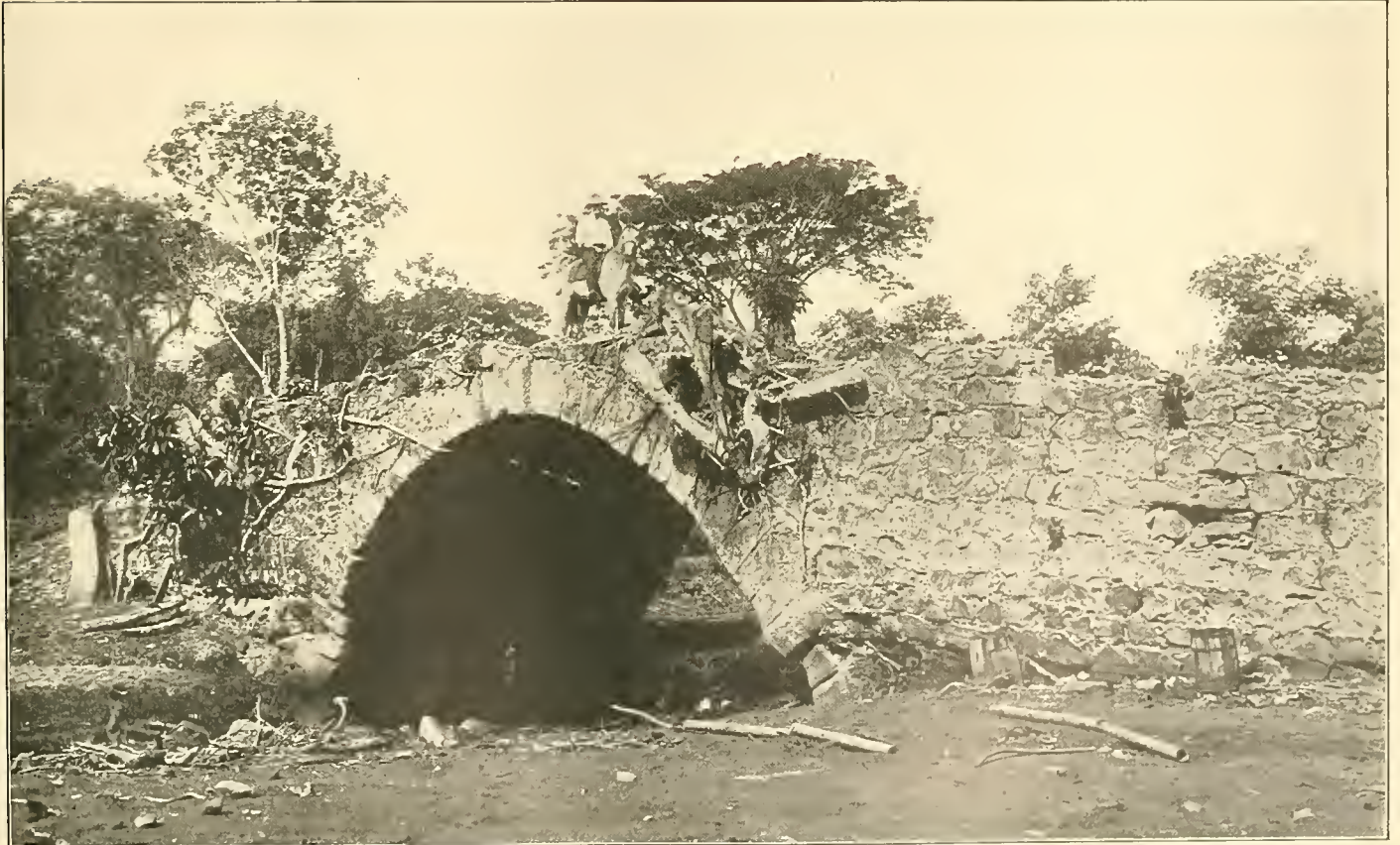
ARCHED BRIDGE AT OLD PANAMA, ALMOST 400 YEARS OLD There was no Horatius to hold this strait path against the invaders
