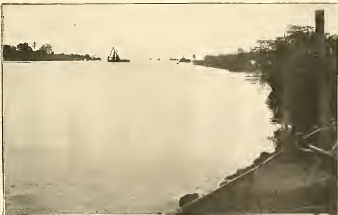
PART OF THE COMPLETED CANAL
