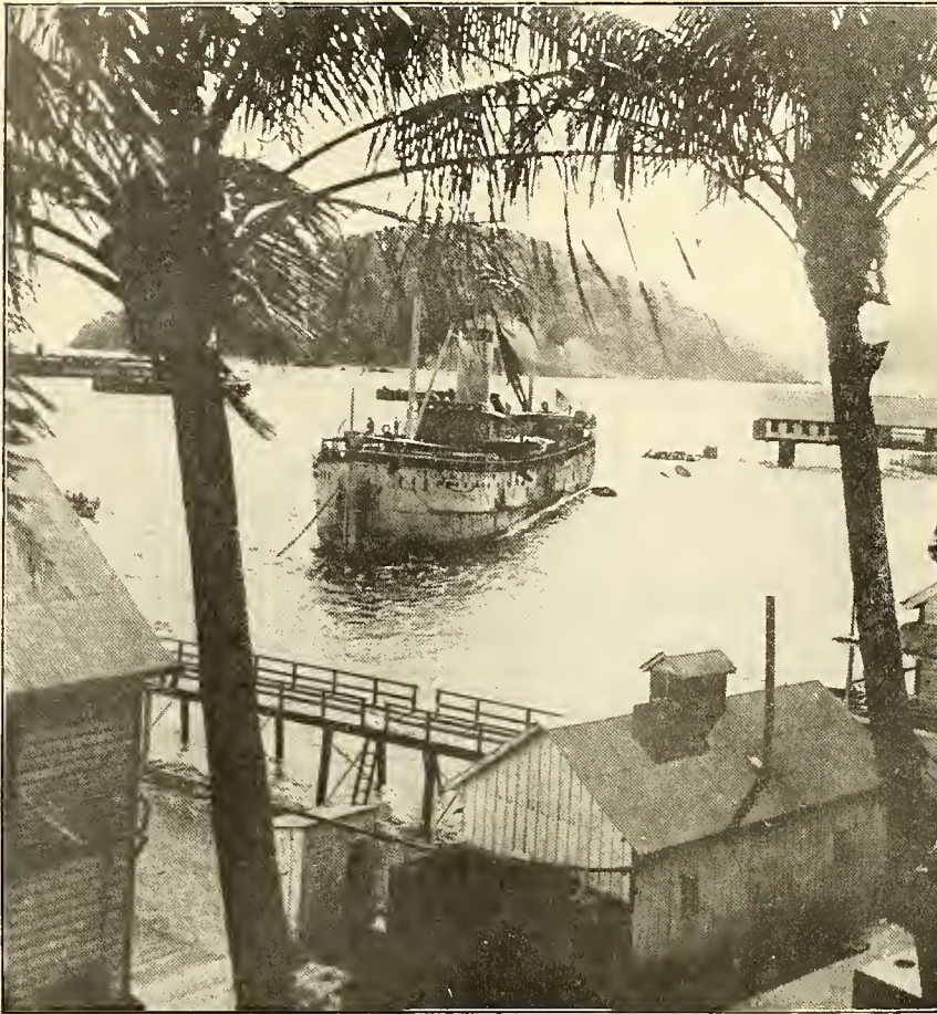
DEEP SEA DREDGE AT BALBOA
