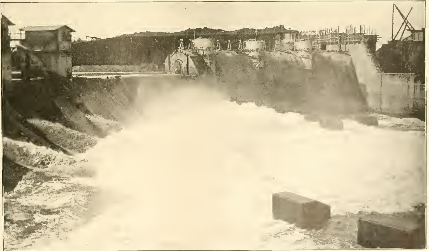
PARTLY COMPLETED SPILLWAY, 1913
