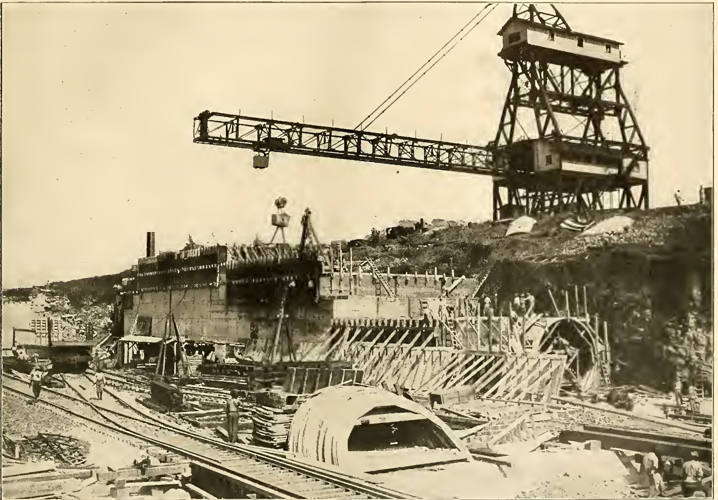
TRAVELING CRANE HANDLING CONCRETE IN LOCK-BUILDING
