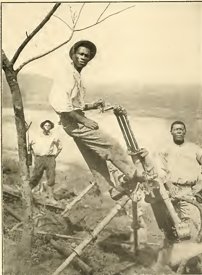
JAMAICANS OPERATING A COMPRESSED AIR DRILL
