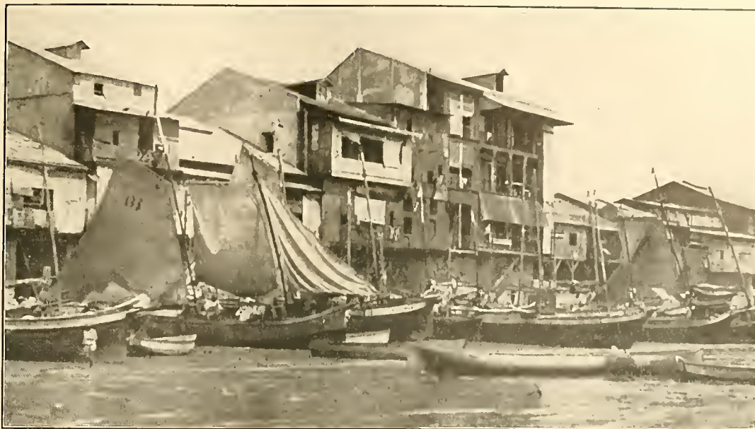
THE PANAMA WATER FRONT
