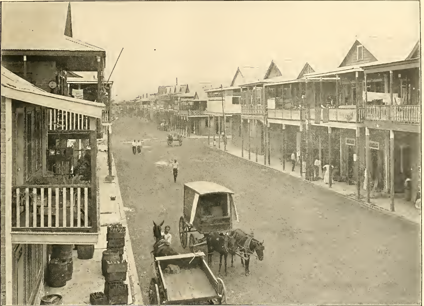
D STREET, COLON, PAVED
