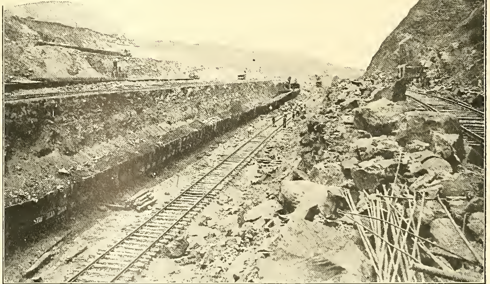
CUTTING AT BASE OF CONTRACTORS HILL
