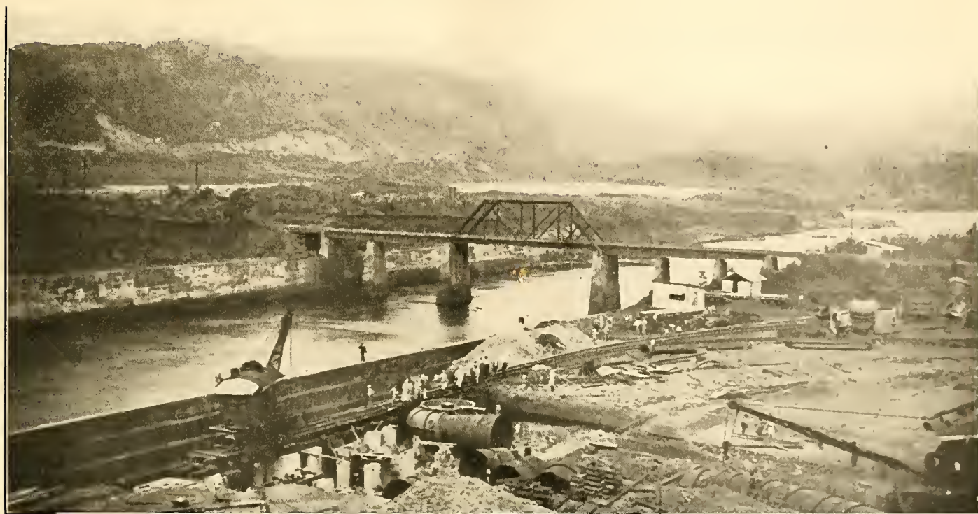
PANAMA RAILROAD BRIDGE ACROSS THE CHAGRES
