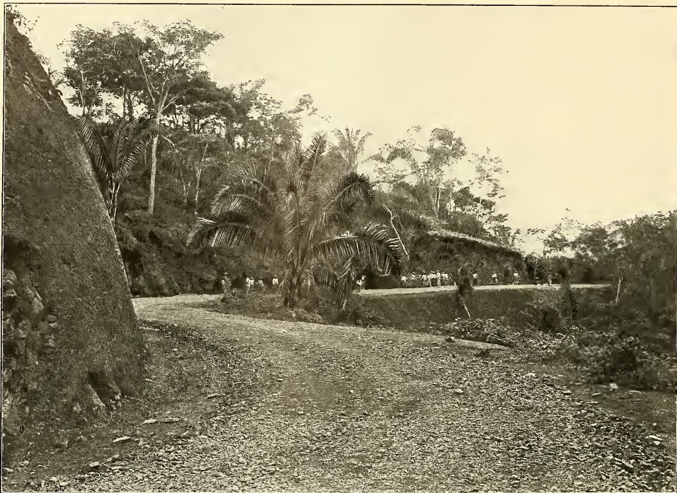
CONVICTS BUILDING A COMMISSION ROAD
